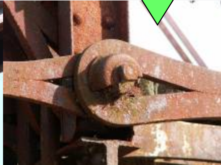
Pinned connections
