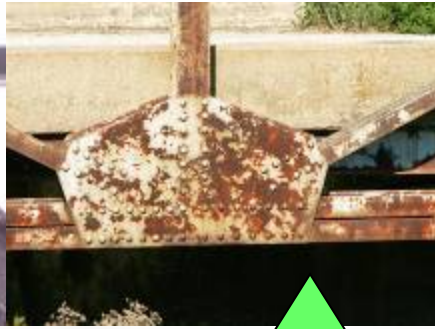
Riveted connections
