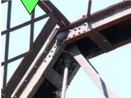
Pinned connections
