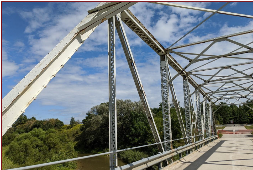
Image 8: Trusses, Guard Rails, and Railings from the West End of the Bridge (Looking Northeast)
