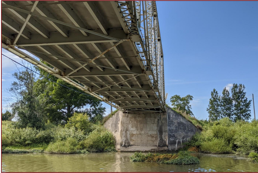
Image 15: North Side of the Bridge
