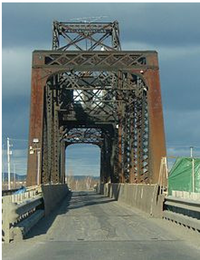
Figure 7: Above – Current bridge deck showing the steel grate deck of the vehicle lane on the left and the pedestrian walk on the right, viewed from the west (photo E. Tumak, Sept. 2013).
