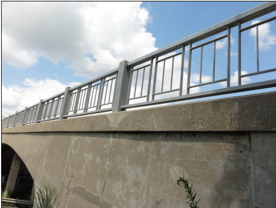
Plate 14: Detail of DHO standard steel railings.
