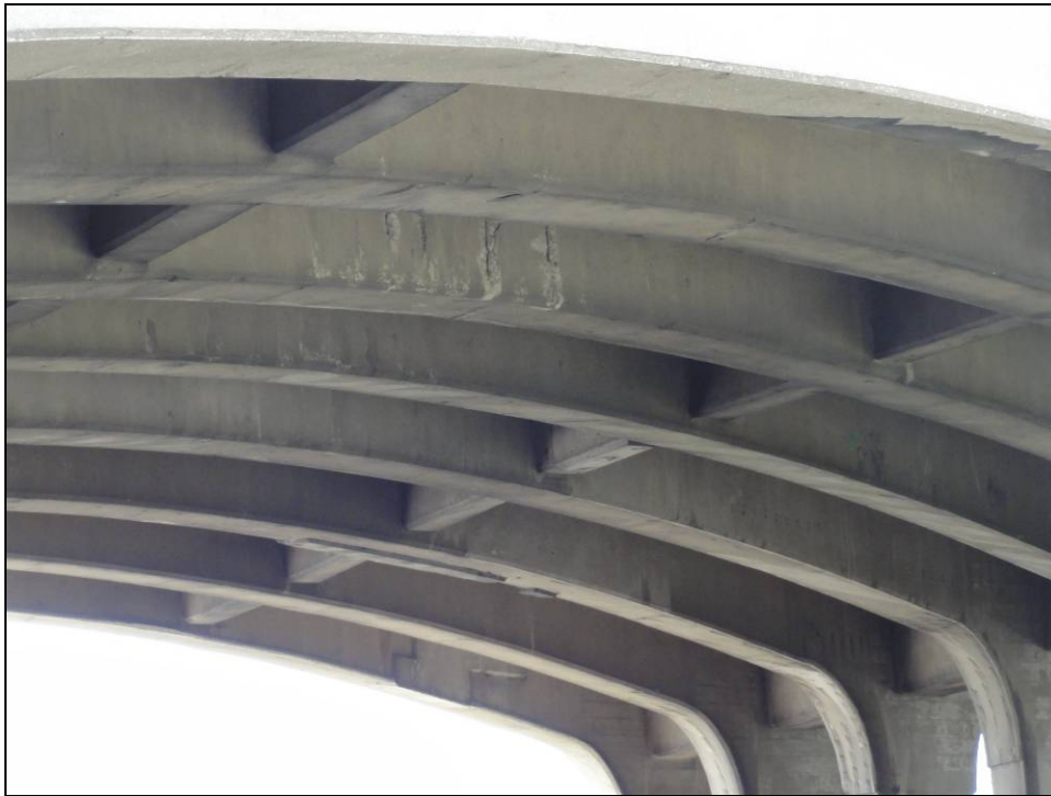
Plate 11: Detail of T-beams.
