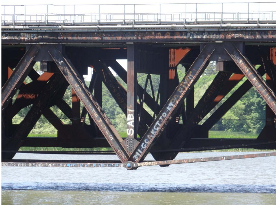
Figure 9-22: Detail of the central section of the deck truss, south elevation.
