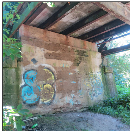
South bridge abutment. Note the 2-ft. (0.61 m) of concrete added in 1908 to raise the bridge.
