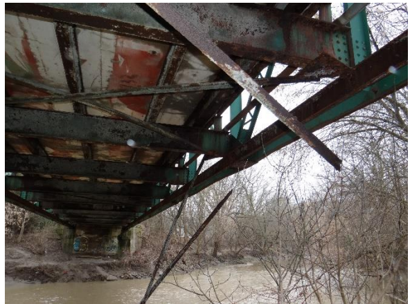
Plate 10: Damaged bracing supporting floor beams in the north portion of the structure, looking southwest
