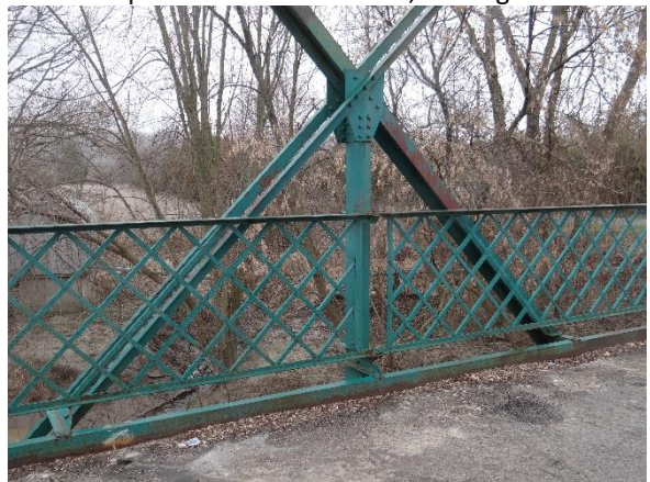
Plate 12: Representative metal lattice railing at deck level.
