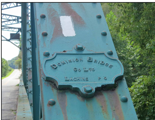
Maker's plaque on the northwest end post, "Dominion Bridge Co. Ltd., Lachine P.Q."
