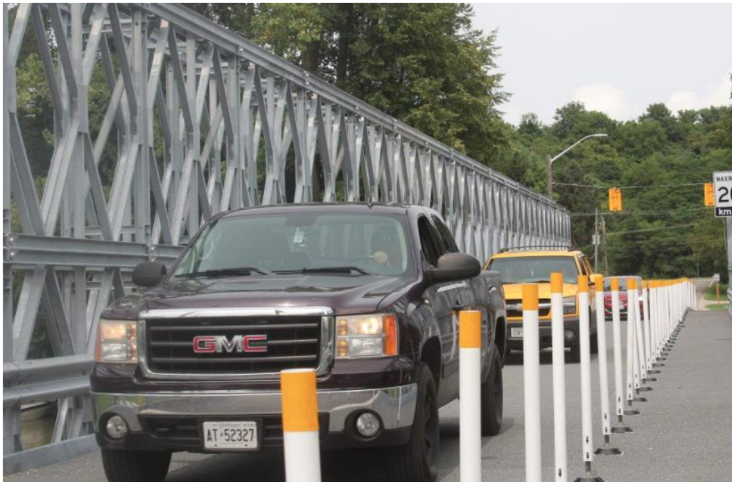
Figure 4: Modular panel bridge in Port Bruce that is anticipated to replace the Meeks Bridge, shown carrying traffic in Port Bruce (Broadley, August 20, et al. 2018)
