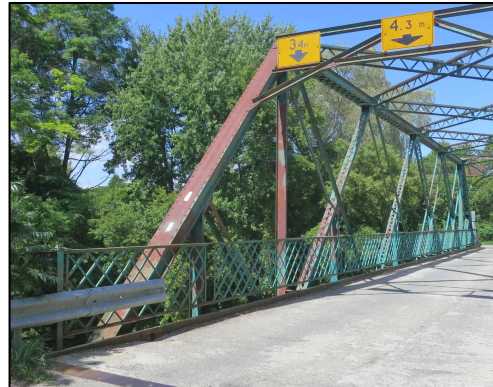
View of the original lattice railing on the west side of Meeks Bridge.
