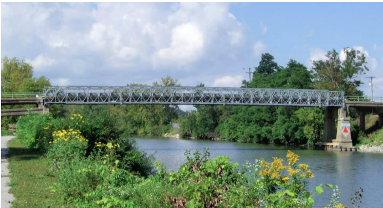
Figure 7: Example of an Acrow truss bridge carrying a roadway in a riverine setting (Image retrieved from Acrow Corporation of America 2020).
