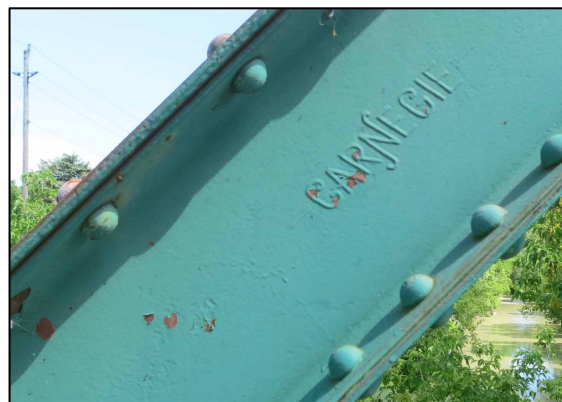
Bridge fabricator mark of "Carnegie" on the side of an end post. One of several similar marks found on the truss structure.
