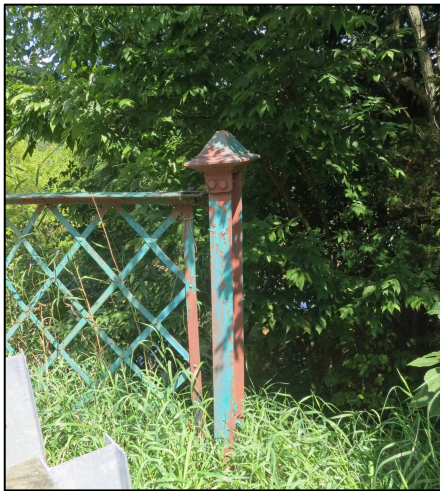
Detail of end post on the southeast bridge corner for the lattice railing. Similarly designed end posts are on all fother corners.
