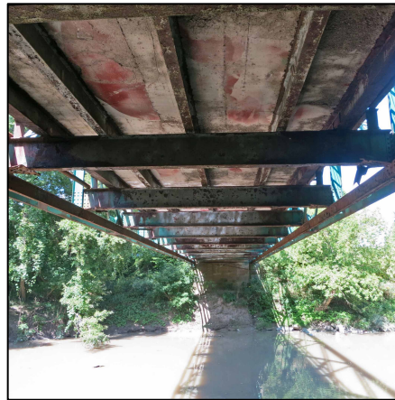
View to north of the steel north to south deck stringers and east to west steel floor beams.
