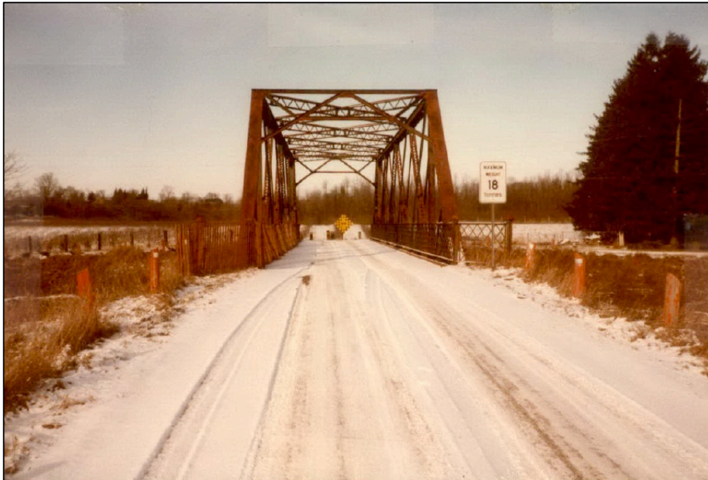
View north to Meeks Bridge on Sparta Line CR 27 showing a weight limit of 18 tonnes. Notice the lack of vegetation on Kettle Creek at the bridge [Elgin County, Meeks Bridge Inspection Report, December 1983].
