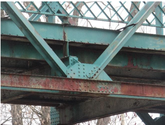
Plate 11: Representative gusset plate with riveted connections to truss diagonals on the east elevation, looking west.
