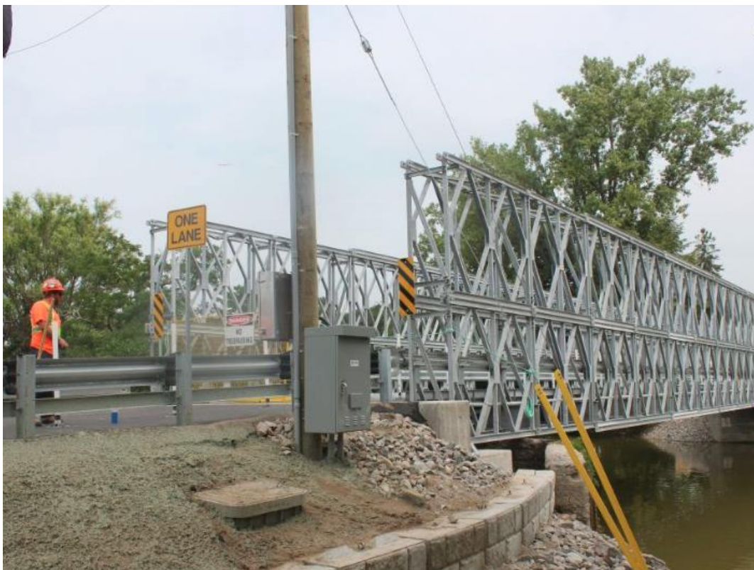
Figure 5: Modular panel bridge in Port Bruce that is anticipated to replace the Meeks Bridge, shown carrying traffic in Port Bruce (Broadley, August 15, et al. 2018)
