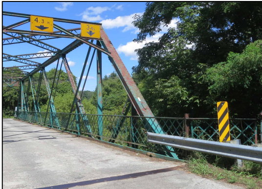
View of the original lattice railing on the east side of Meeks Bridge.
