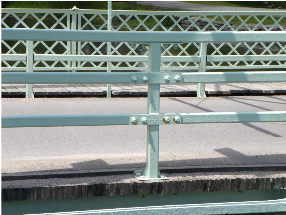
Plate 15: Deck railings in foreground, lattice pedestrian railing in background and wood deck with asphalt paving.
