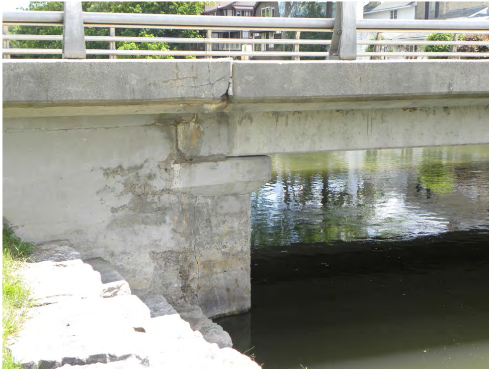
Plate 22: Abutment and wing walls showing original 1912 abutment and 1971 additions.
