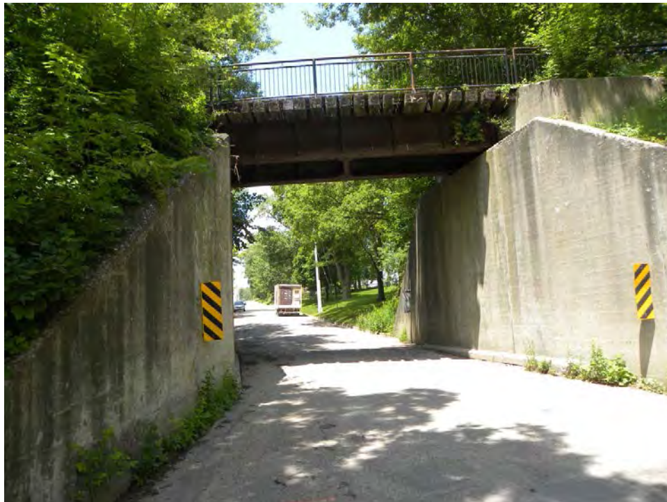
Plate 25: Emily Street Underpass, showing steel plate girder span, abutment, wing walls, earth embankment and deck.
