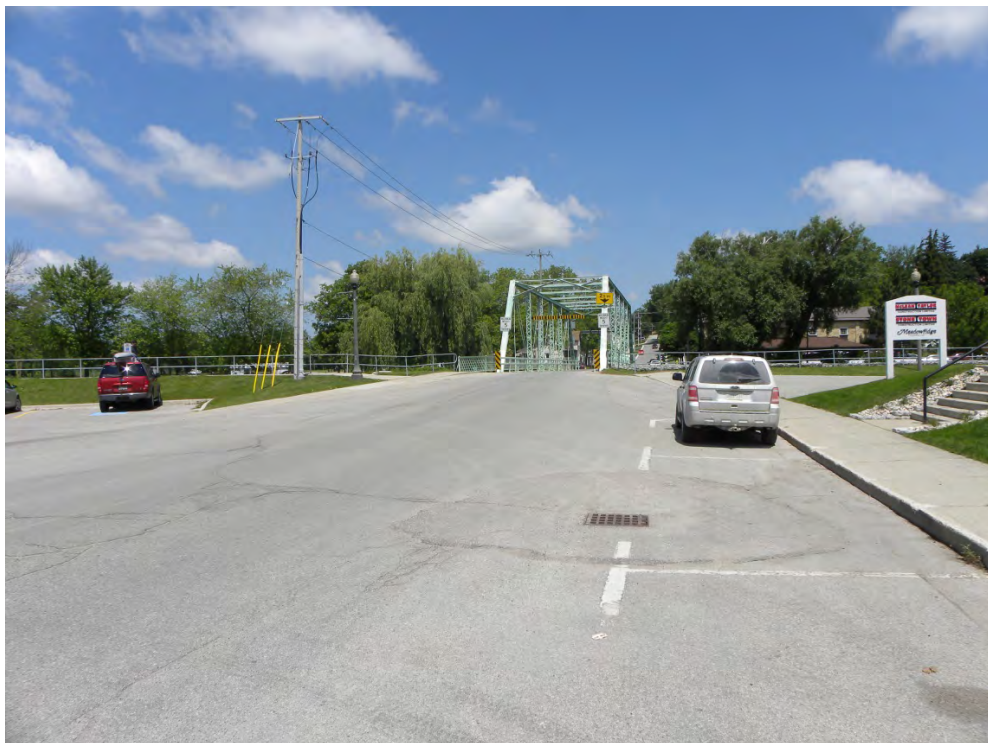
Plate 16: Water Street approach to bridge showing raise in grade up to bridge abutments
