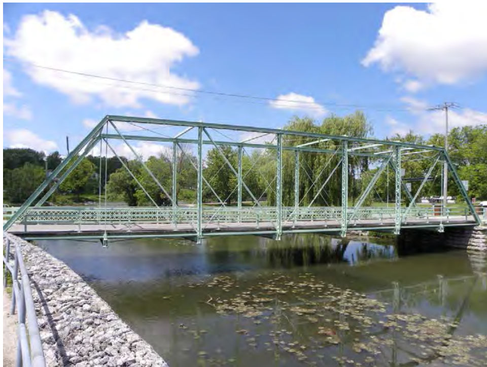
Plate 9: Water Street Bridge, east side, looking west and showing the gabion baskets along the south bank. The Thames River is barely visible in the distance.
