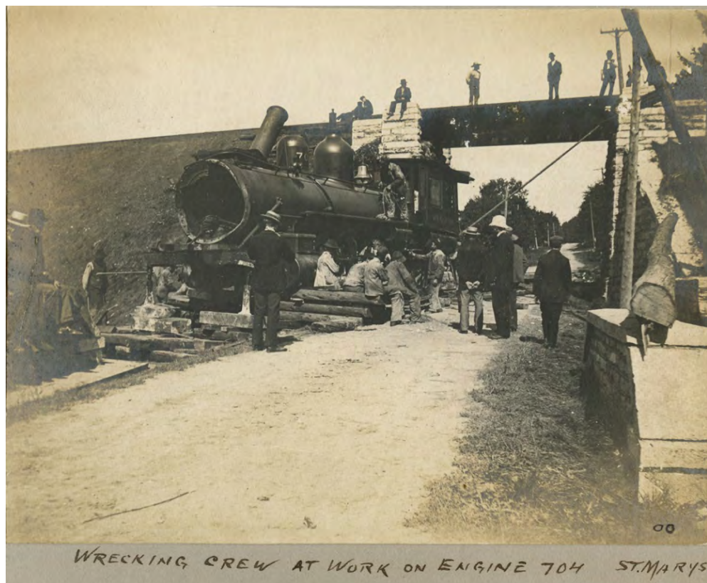
Plate 7: Emily Street Underpass 1905, showing stone abutments, wing walls, and iron plate girder (St. Marys Museum, reesor041).
