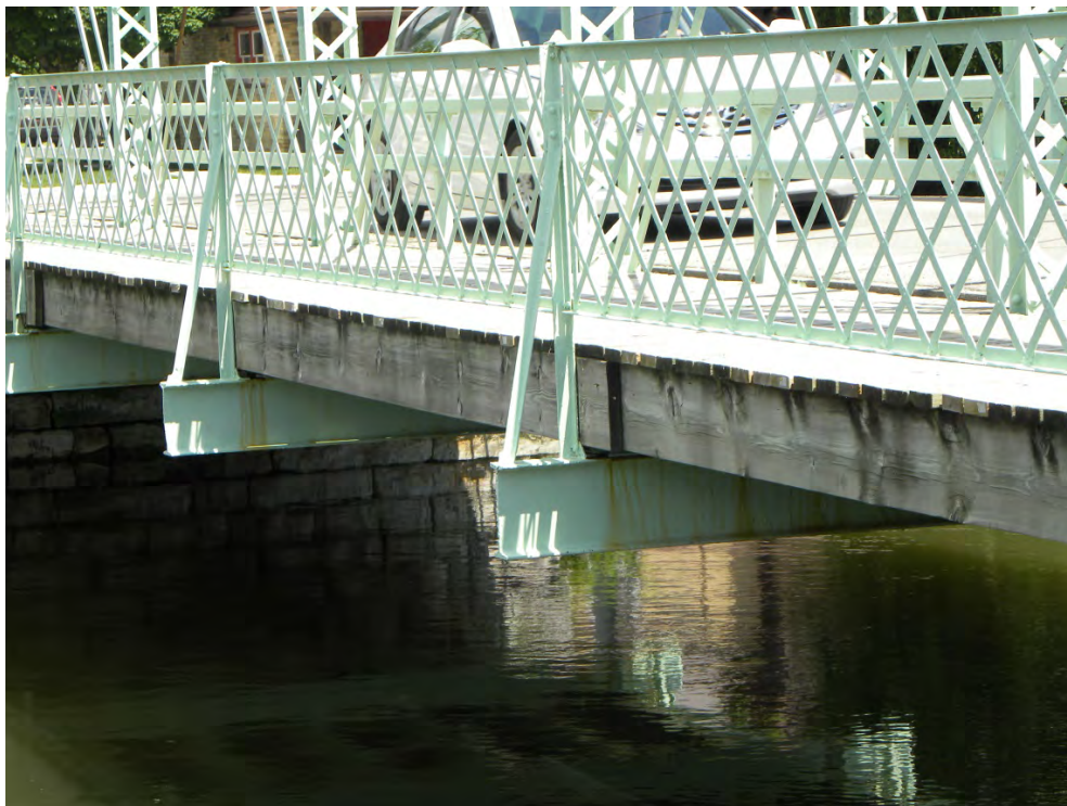
Plate 14: Walkway resting on crossbeams and posts welded to cross beams
