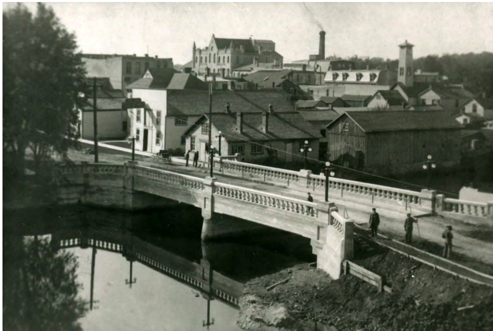
Plate 4: Wellington Street Bridge 1912 Construction showing decorative balustrades, wing walls and panels (St Marys Museum, 1705ph).
