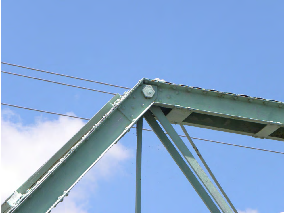
Plate 11: Structural pin connection between top chord, diagonals and inclined end post.
