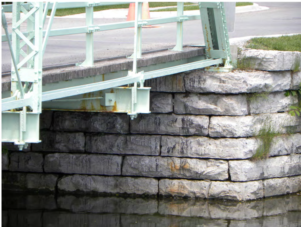
Plate 12: North end abutment, showing pitch-faced squared limestone
