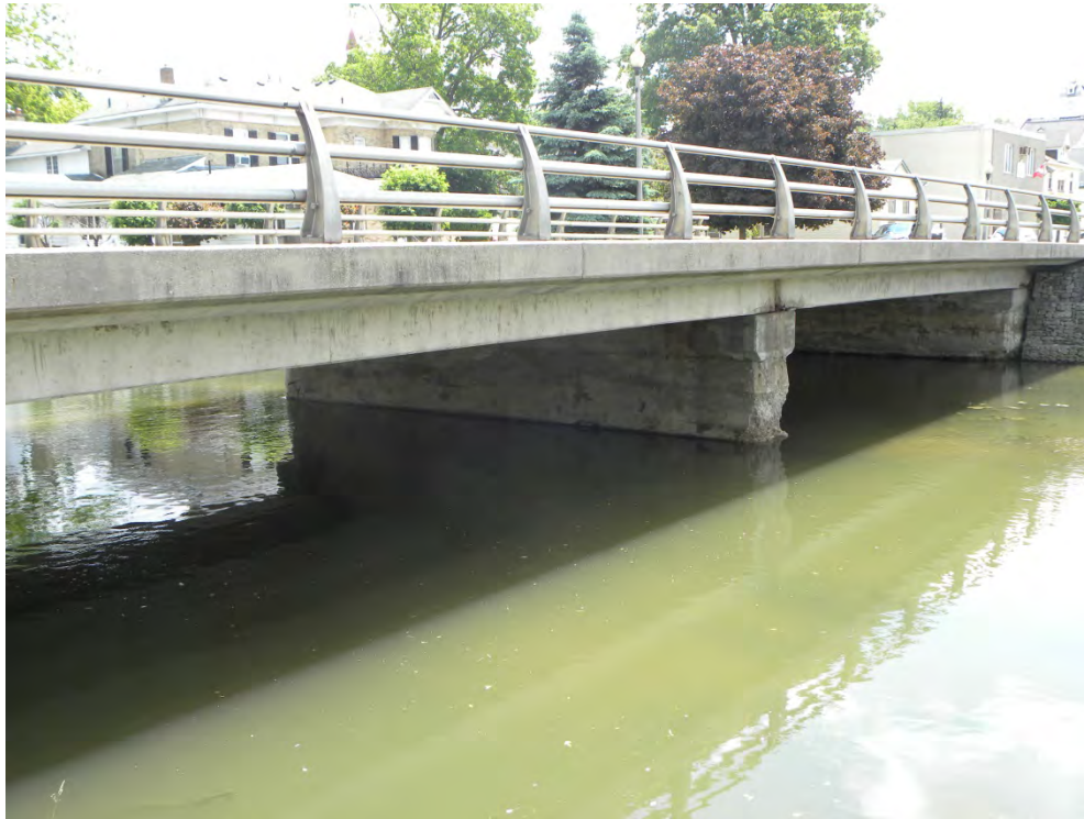
Plate 6 Wellington Street Bridge, west side showing the concrete centre pier of the 1912 bridge.
