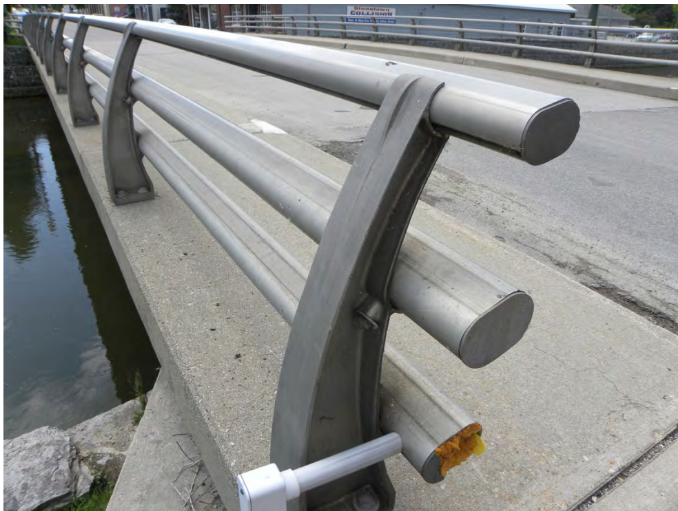
Plate 23: Railings showing cast posts and extruded aluminium rails
