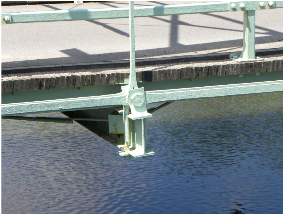
Plate 13: Substructure showing paved timber deck, bottom chord, cross bream, and structural pin connection
