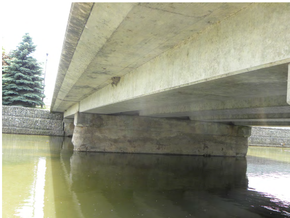
Plate 19: Original 1912 pier supporting 1971 concrete box girders, deck replacement
