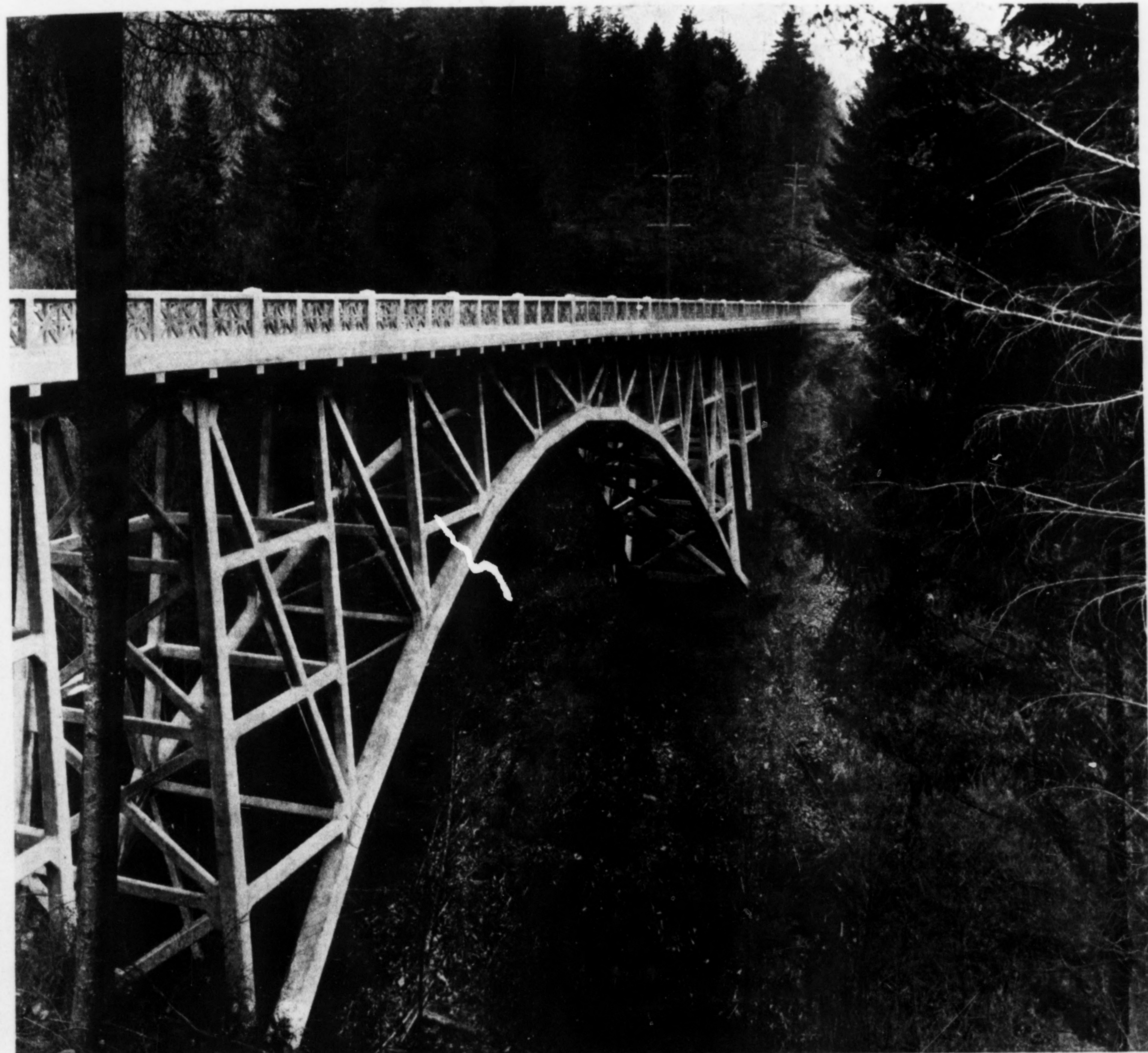
Alexander Avenue Viaduct, Portland, Oregon
