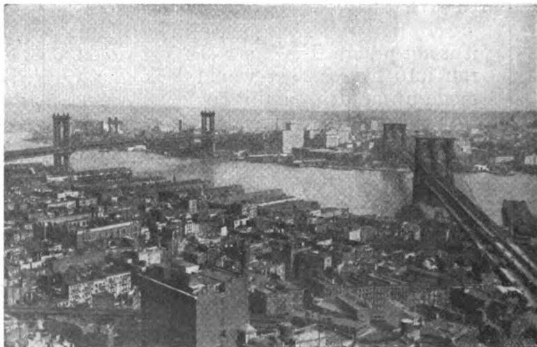
At the right is Brooklyn Bridge, built by Roebling years ago. Overloaded far beyond the capacity for which it was intended, it threatened to collapse in 1901, but was repaired by Lindenthal and is still in service. At the left is Manhattan Bridge. Lindenthal designed it originally; but, owing to a change in the city administration, it was built by other engineers, who altered the plans
