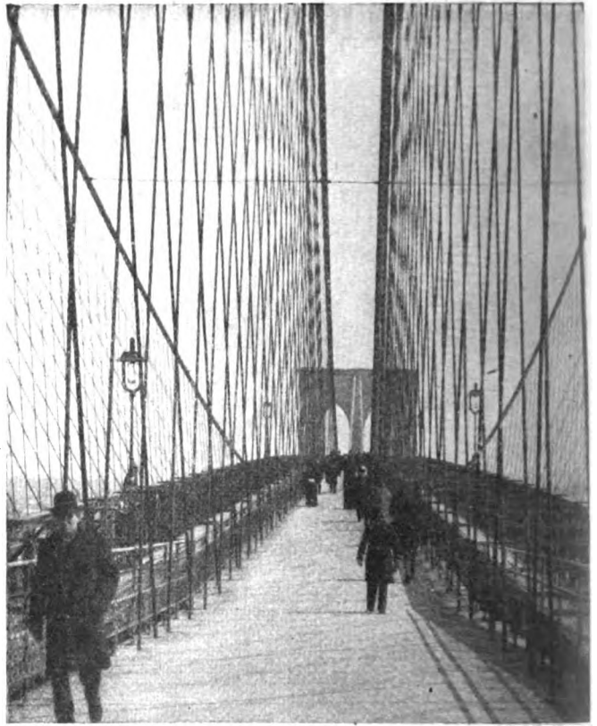
When Brooklyn Bridge was built, 1870-1883, it had the longest single span in the world, 1,595 feet in length and about 150 feet above the water. It has double tracks for elevated trains, a wide roadway for vehicles, two tracks for surface cars, and a promenade, shown above, for pedestrians
