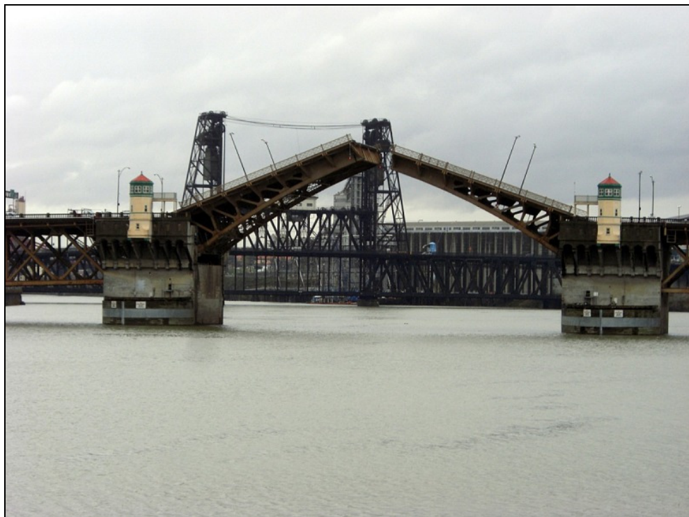
Photo 6 of 6: (OR_MultnomahCounty_WillametteHwyBridgesMPD_BurnsideBridge_0006) Downstream view, showing bascule in operation (Steel bridge in distance)
