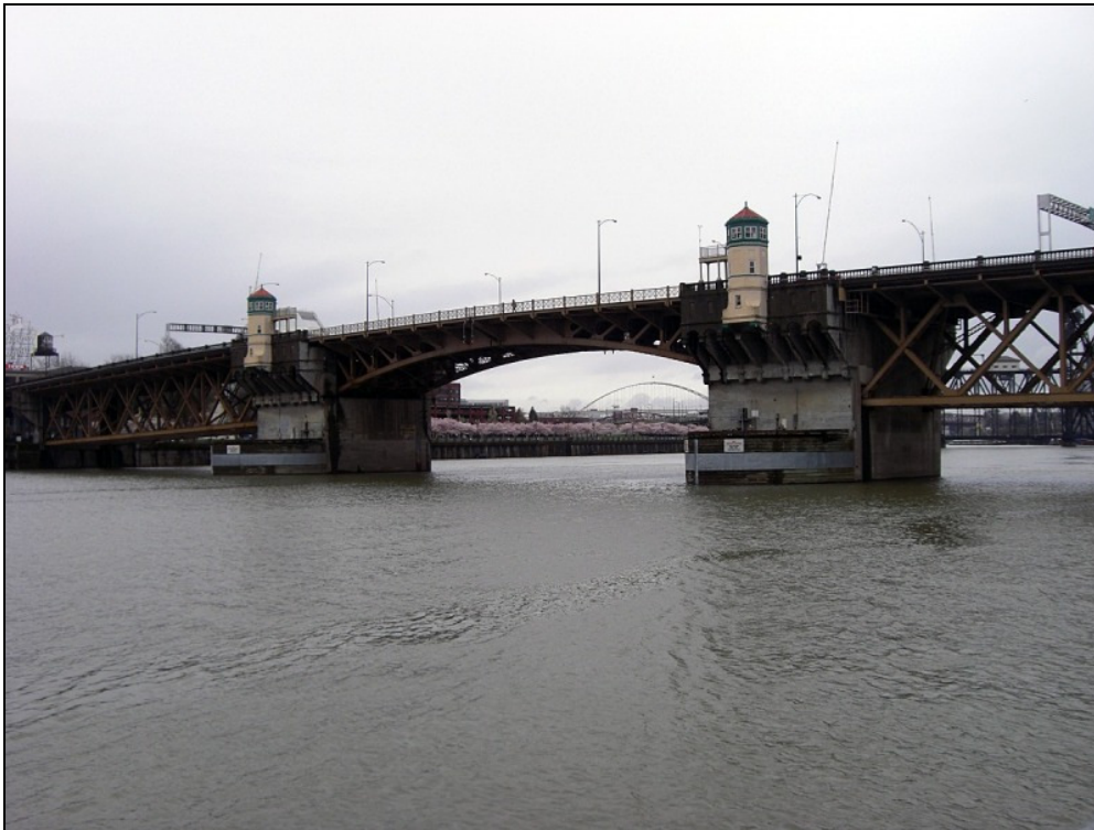
Photo 2 of 6: (OR_MultnomahCounty_WillametteHwyBridgesMPD_BurnsideBridge_0002) Upstream view, looking NW, from Vera Katz Esplanade
