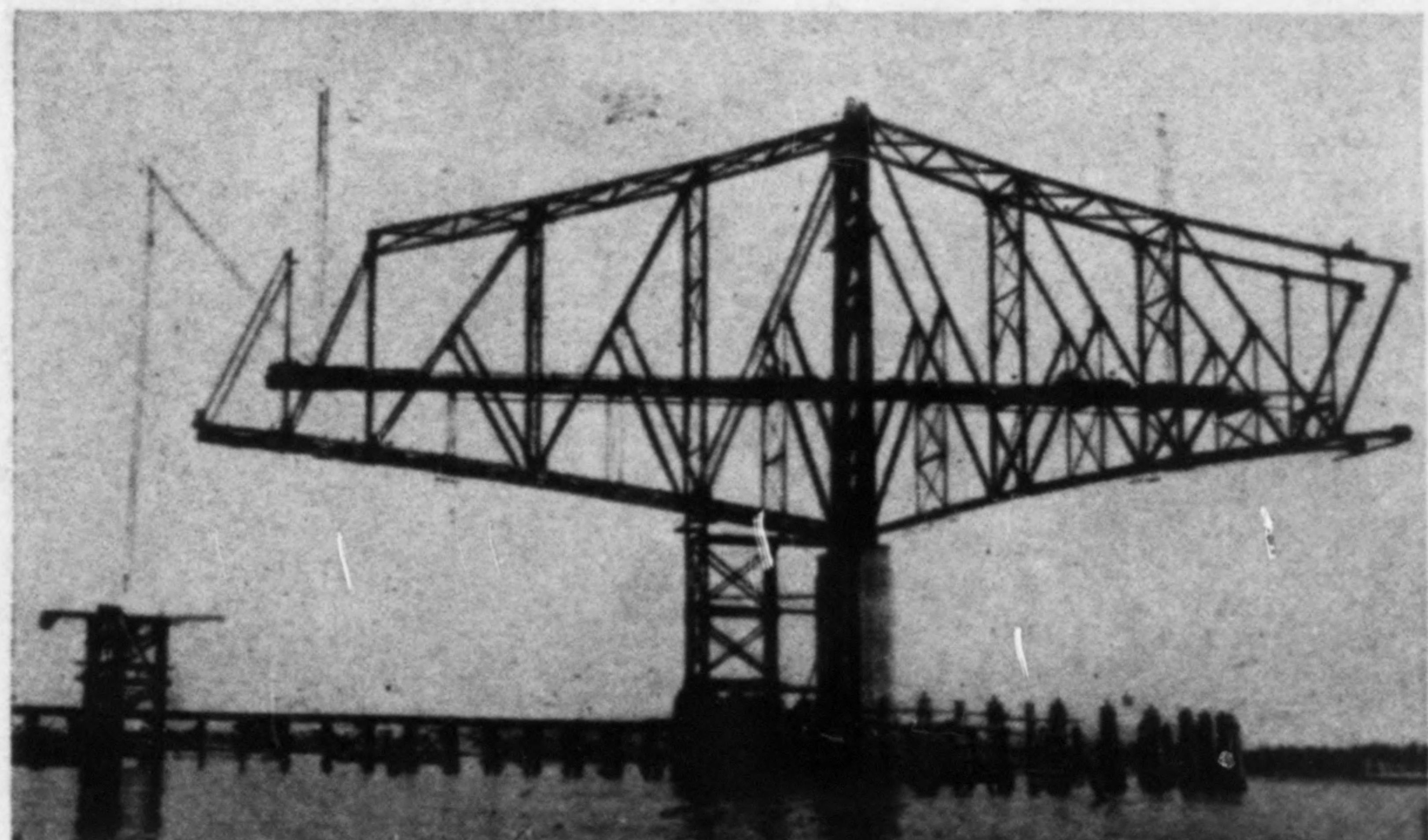
FIG. 5—TWO STAGES of balanced erection of cantilever bridge using two falsework bents equipped with hydraulic jacks under the anchor span.
