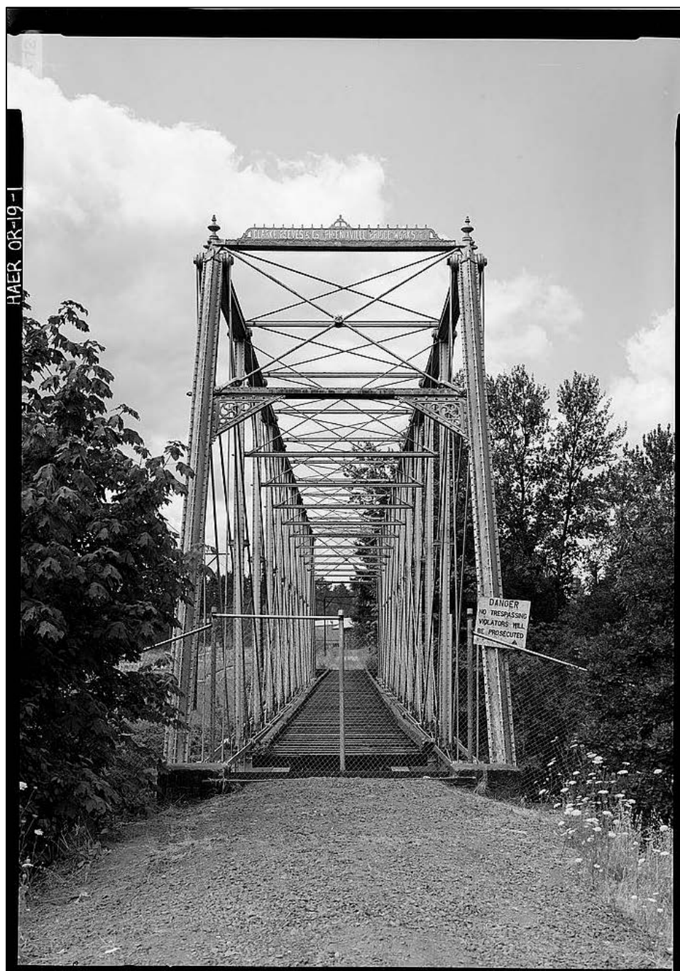
Figure 15: Hayden Bridge, Springfield, showing Phoenix Bridge (Clark & Reeves) Portal Screen, Eastern Portland, Looking West (HABS Photo, ORE-20, SPRIF---1), 1992
