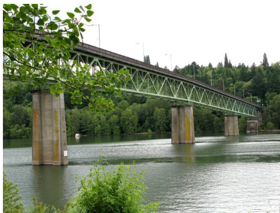
Fig. 5. North Elevation, Warren Truss. Rittergrup Photo
