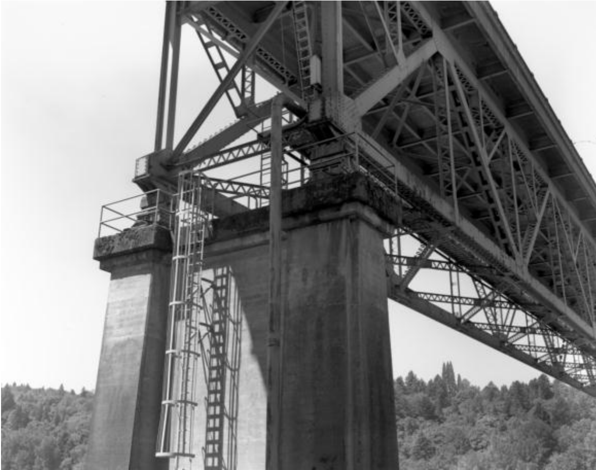
HAER OR-103-30 Detail view of reinforced concrete pier and east end of steel truss structure (2011 combined view of HAER OR-103-11 and OR-103-12 taken in 1999).
