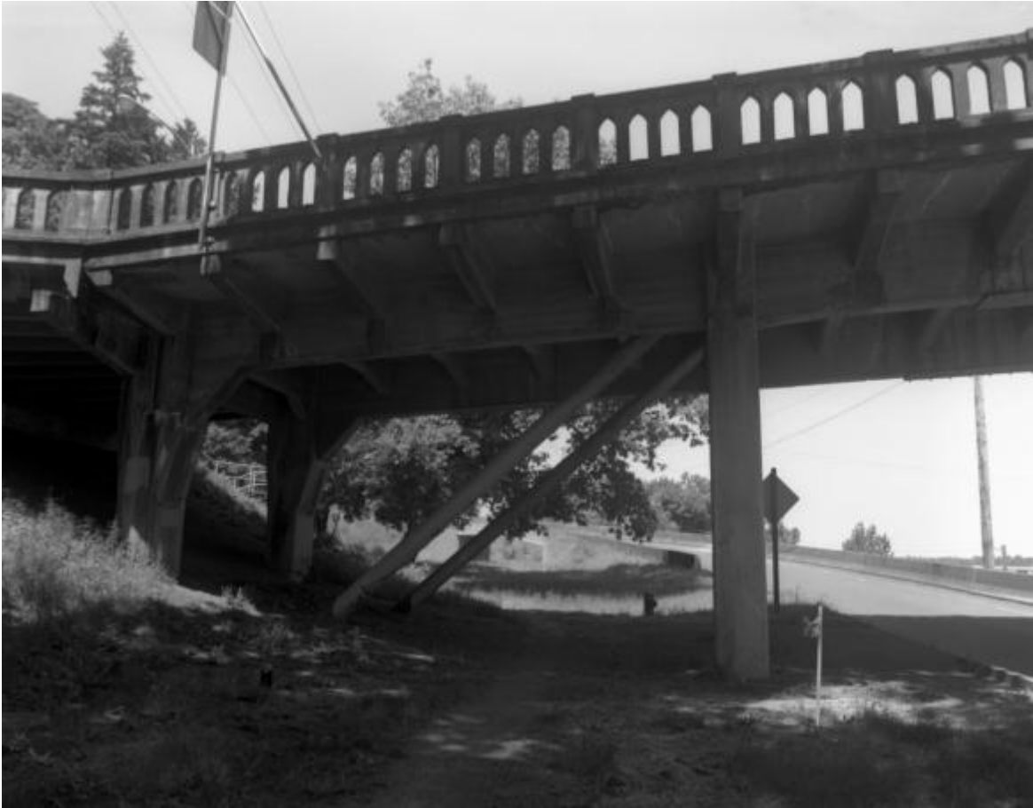
HAER OR-103-31 Detail view of reinforced concrete approach span with bracing at west end of the Sellwood Bridge (2011 view of HAER OR-103-14 taken in 1999).
