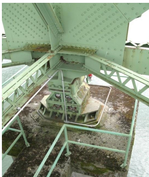
Fig. 9. Bearing, Pier 19.
