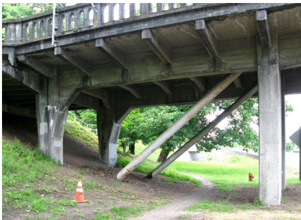
Fig. 31. Bracing at Span 27
