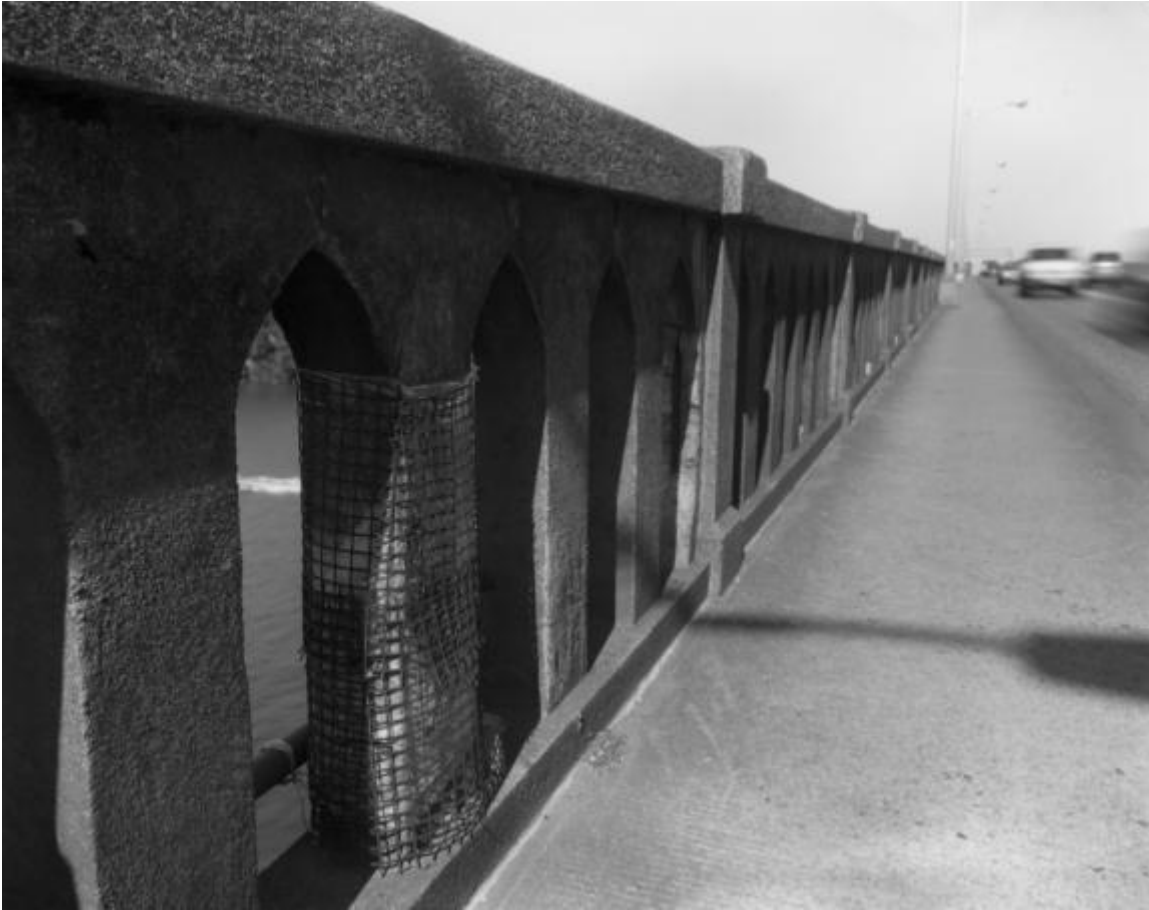
HAER OR-103-32 Detail view showing temporary repair of Sellwood Bridge precast concrete guard rail baluster (see HAER OR-103-16 for 1999 view of intact railing).
