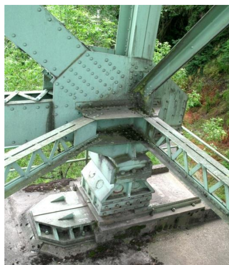
Fig. 12. Bearing, Pier 21
