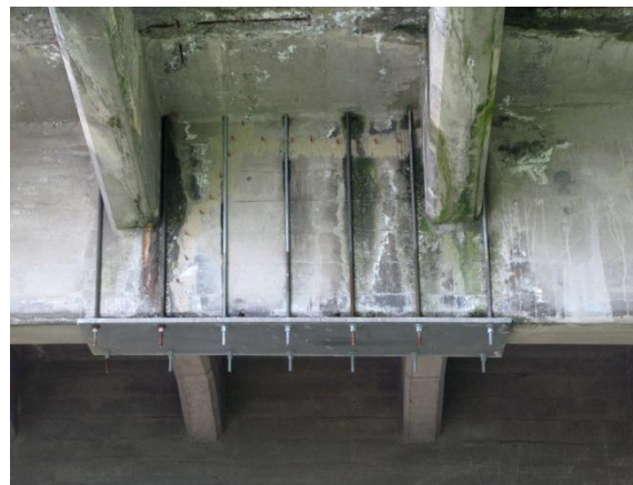
Fig. 32. Span 27 Reinforcement
