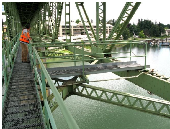
Fig. 8. Maintenance Catwalk Rittergrup Photo
