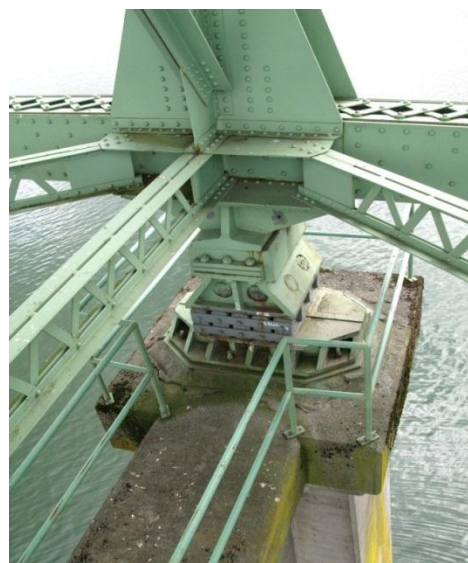
Fig. 10. Bearing, Pier 18
