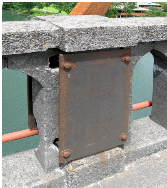
Fig. 24. Connector Plate
