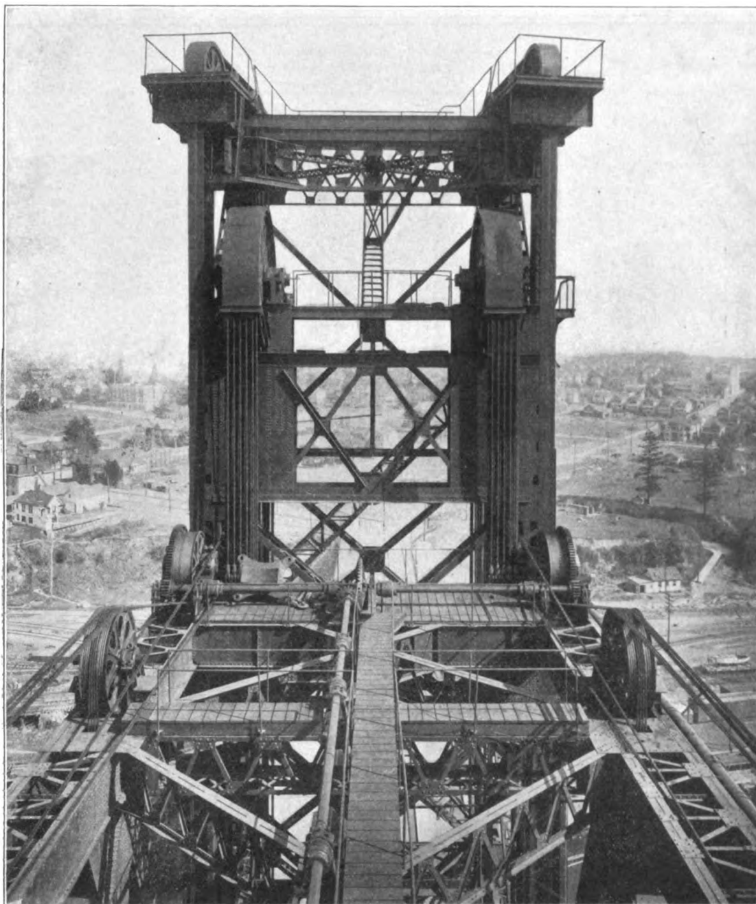
New O.-W. R. R. & N. Co. Lift Bridge at Portland, Ore. Fig. 4—Top View of Tower and Lifting Pulleys.
