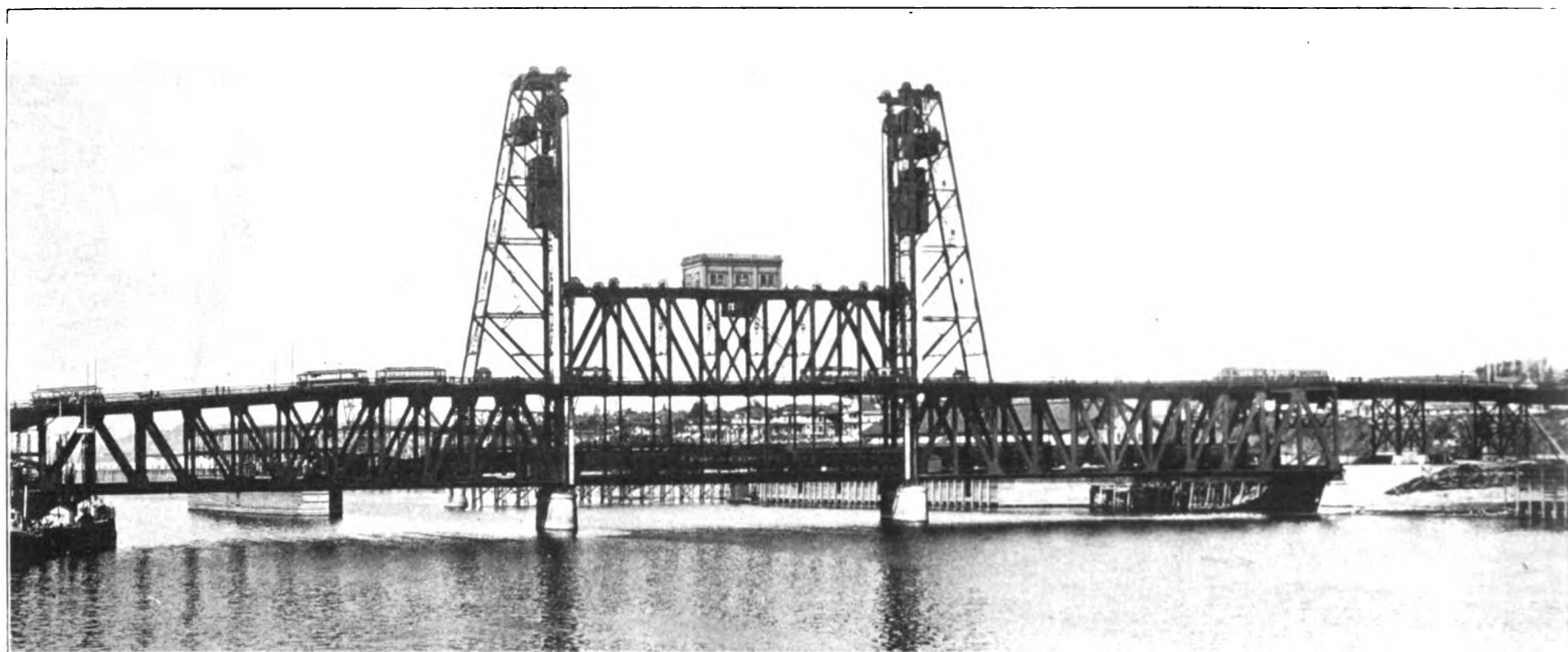
New O.-W. R. R. & N. Co. Lift Bridge at Portland, Ore. Fig. 1—Upper and Lower Decks in Normal Position.
