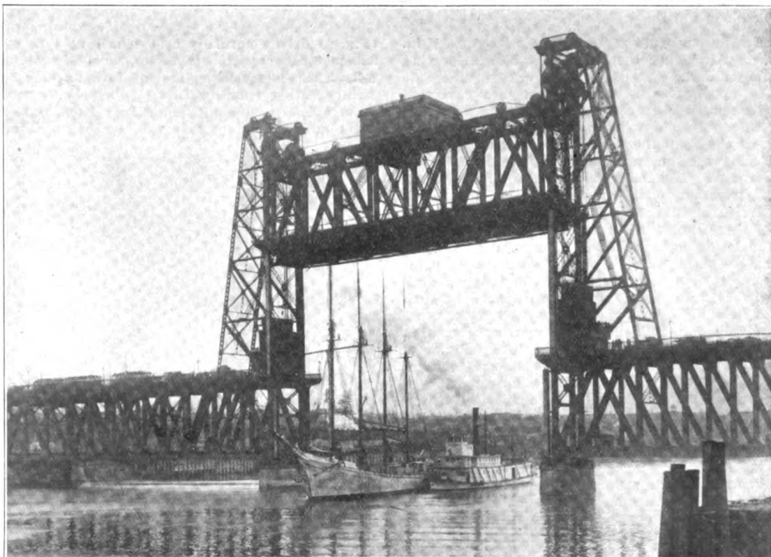
New O.-W. R. R. & N. Co. Lift Bridge at Portland, Ore. Fig. 3—Upper and Lower Decks Telescoped and Lifted.
