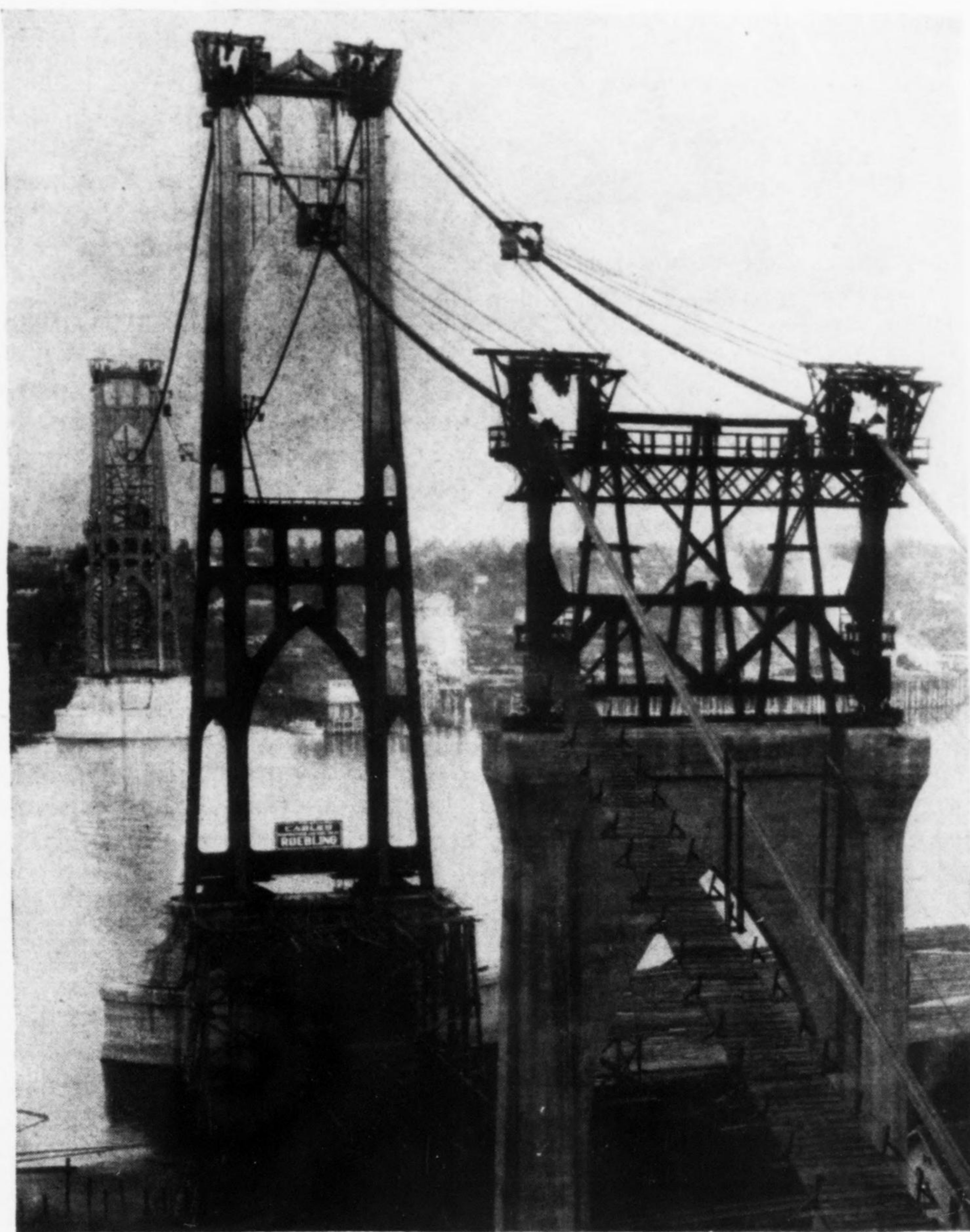
Fig. 4—Layout of cable-stringing operations
