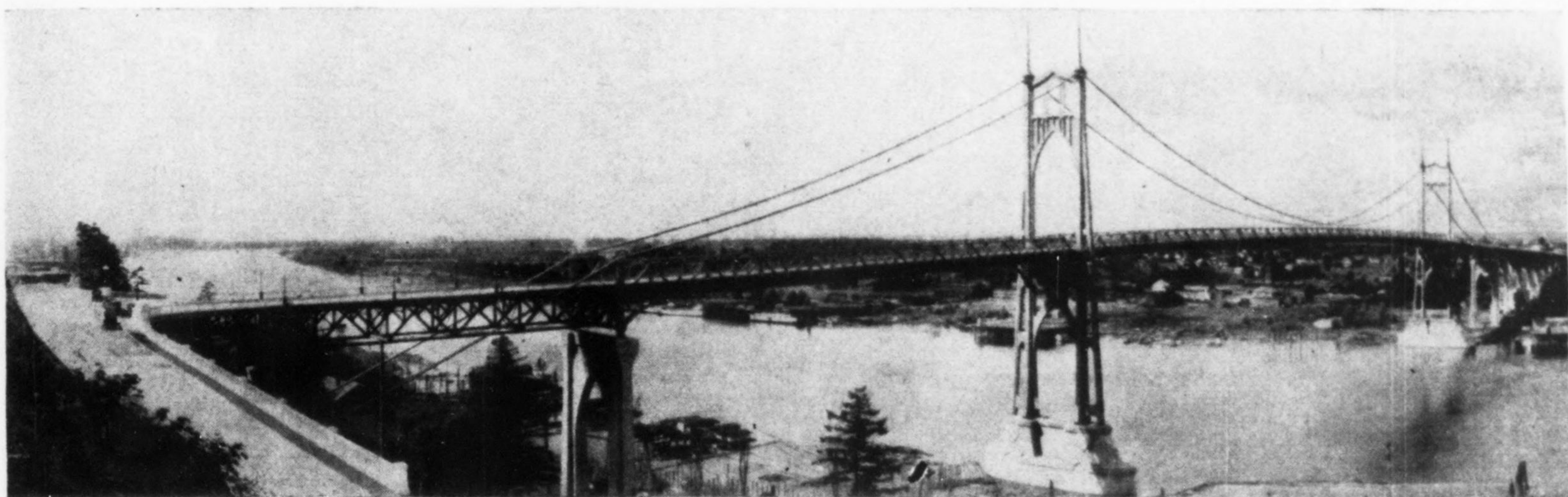
•Fig. 1—St. Johns bridge, Portland, Ore., establishes a record span of 1,207 ft. for rope-strand cable type
