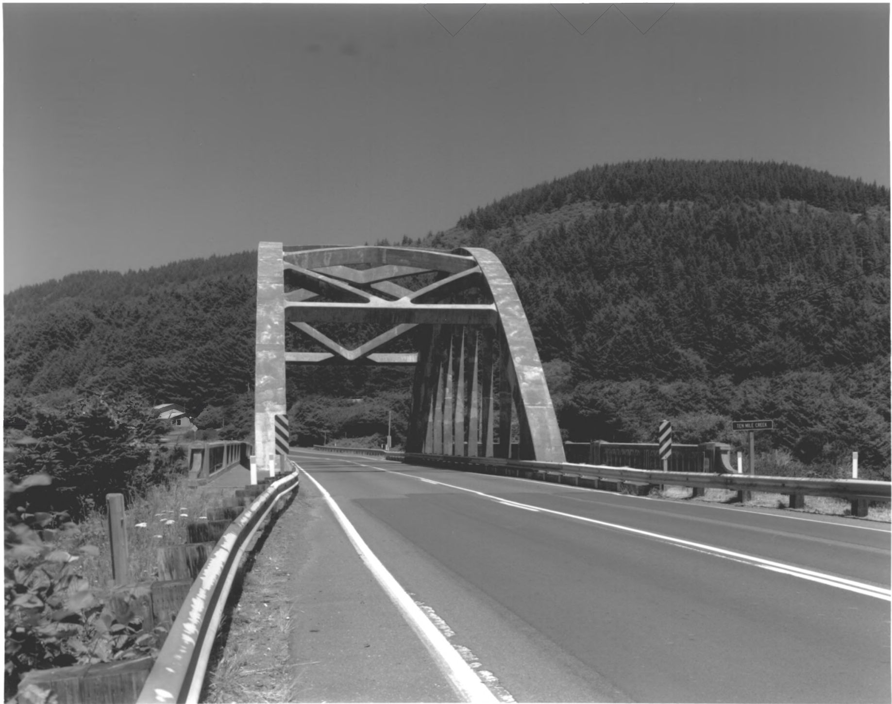
TENMILE CREEK BRIDGE, YACHTS VICINITY, OREGON #1
