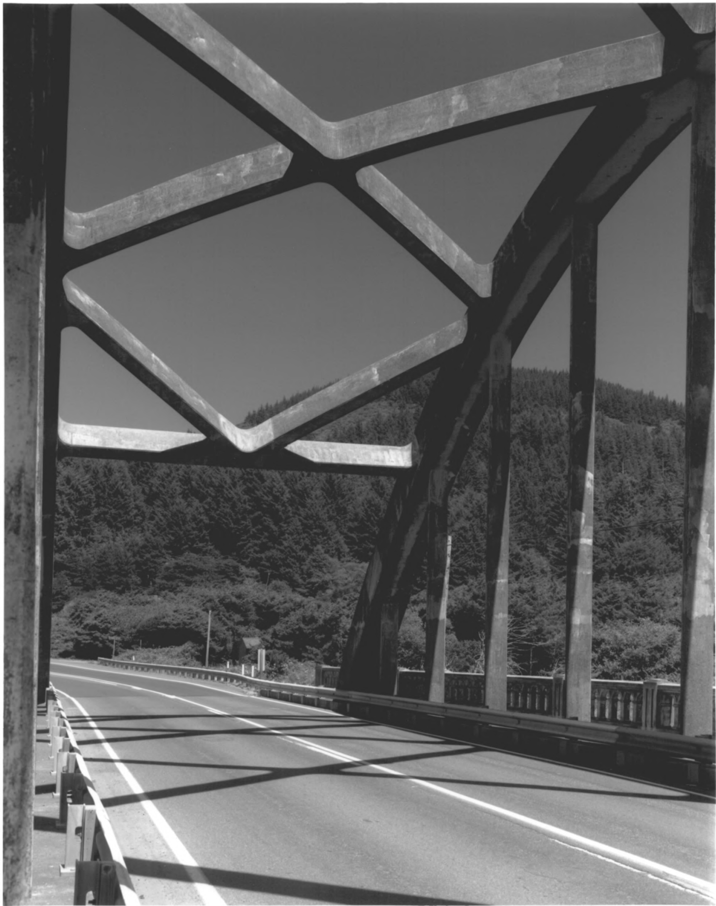
TENMILE CREEK BRIDGE, YACHTS VICINITY, OREGON #2
