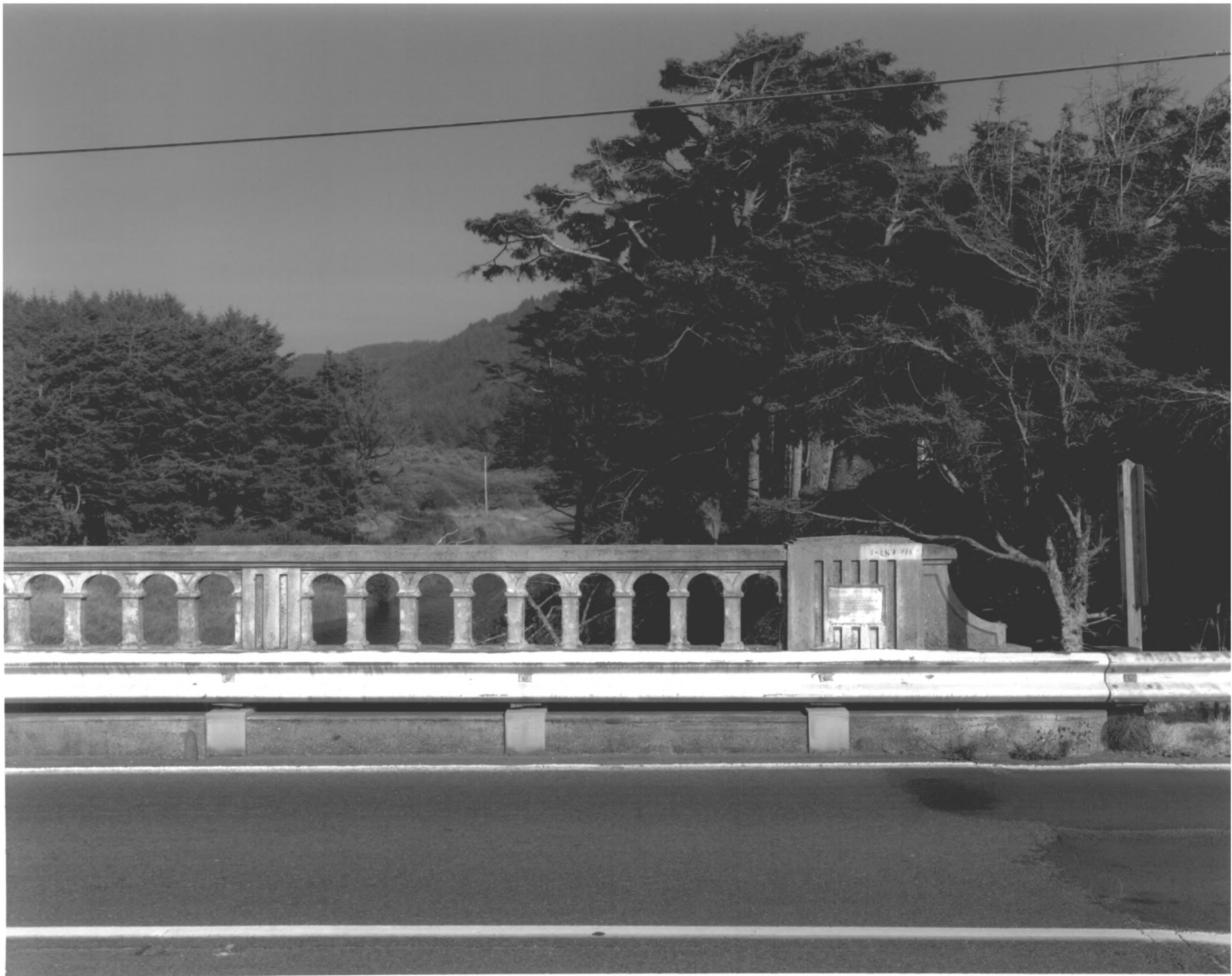
TEN MILE CREEK BRIDGE, YACHTS VICINITY, OREGON # 5
