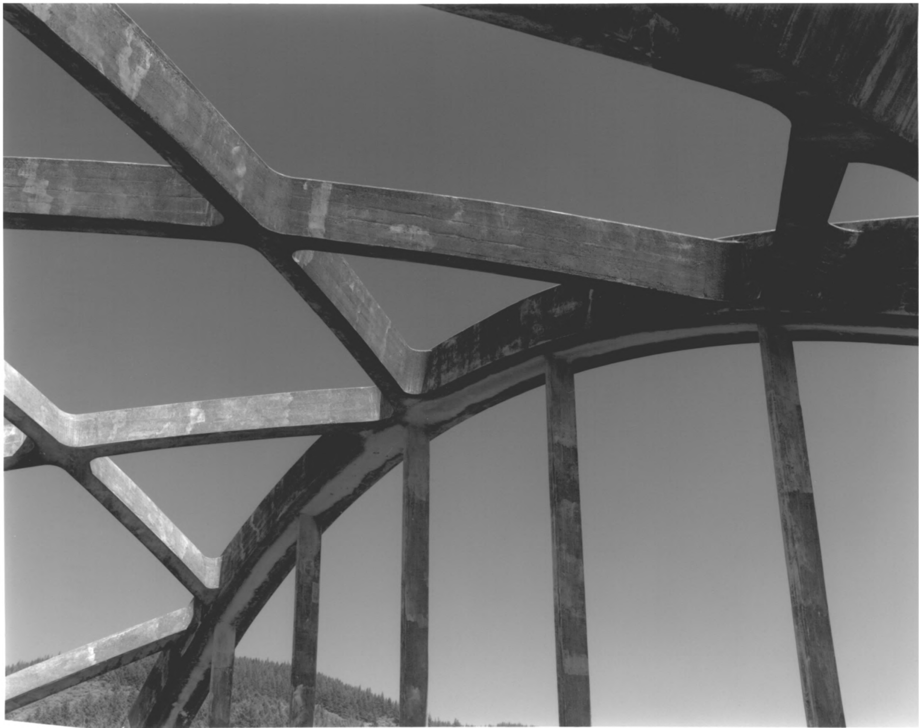
TENMILE CREEK BRIDGE, YACHTS VICINITY, OREGON #3
