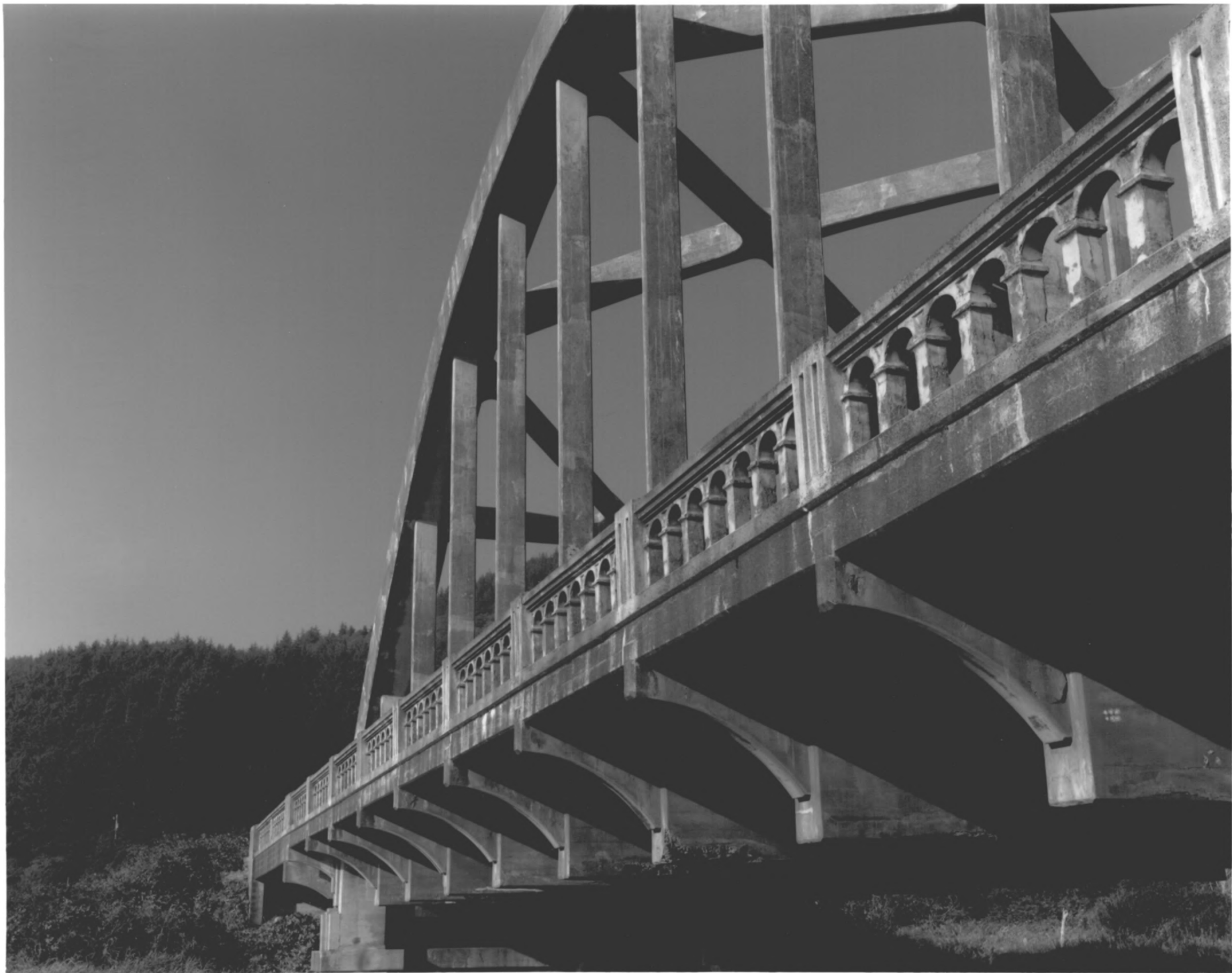
TENMILE CREEK BRIDGE, YACHATS VICINITY, OREGON #A
