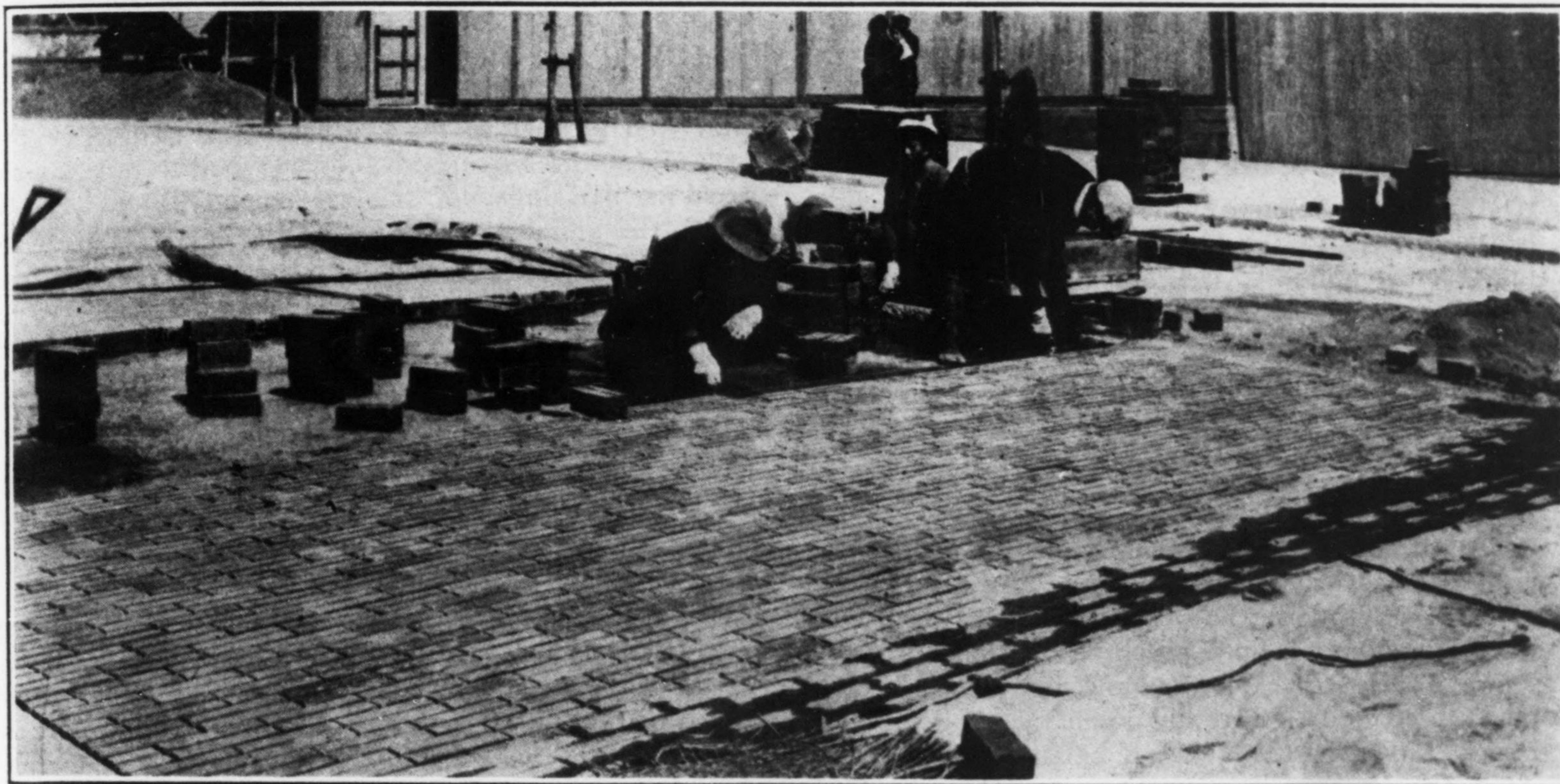
JAPANESE PAVEMENT LAYING GROOVED BRICK PAVEMENT IN TOKYO
