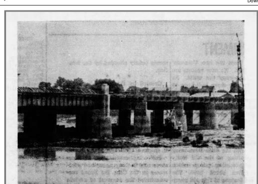
BLACK RIVER BRIDGE — The construction of the highway bridge over Black river near the west end of Scott avenue is nearing completion. This structure will ultimately carry by-pass traffic between M-21 (Lapeer Ave.) and M-51 (Pine Grove Ave.) and the Blue Water Bridge. The total cost of the bridge including grading and drainage work is estimated at approximately \$850,000, of which the City's share is \$50,000.
