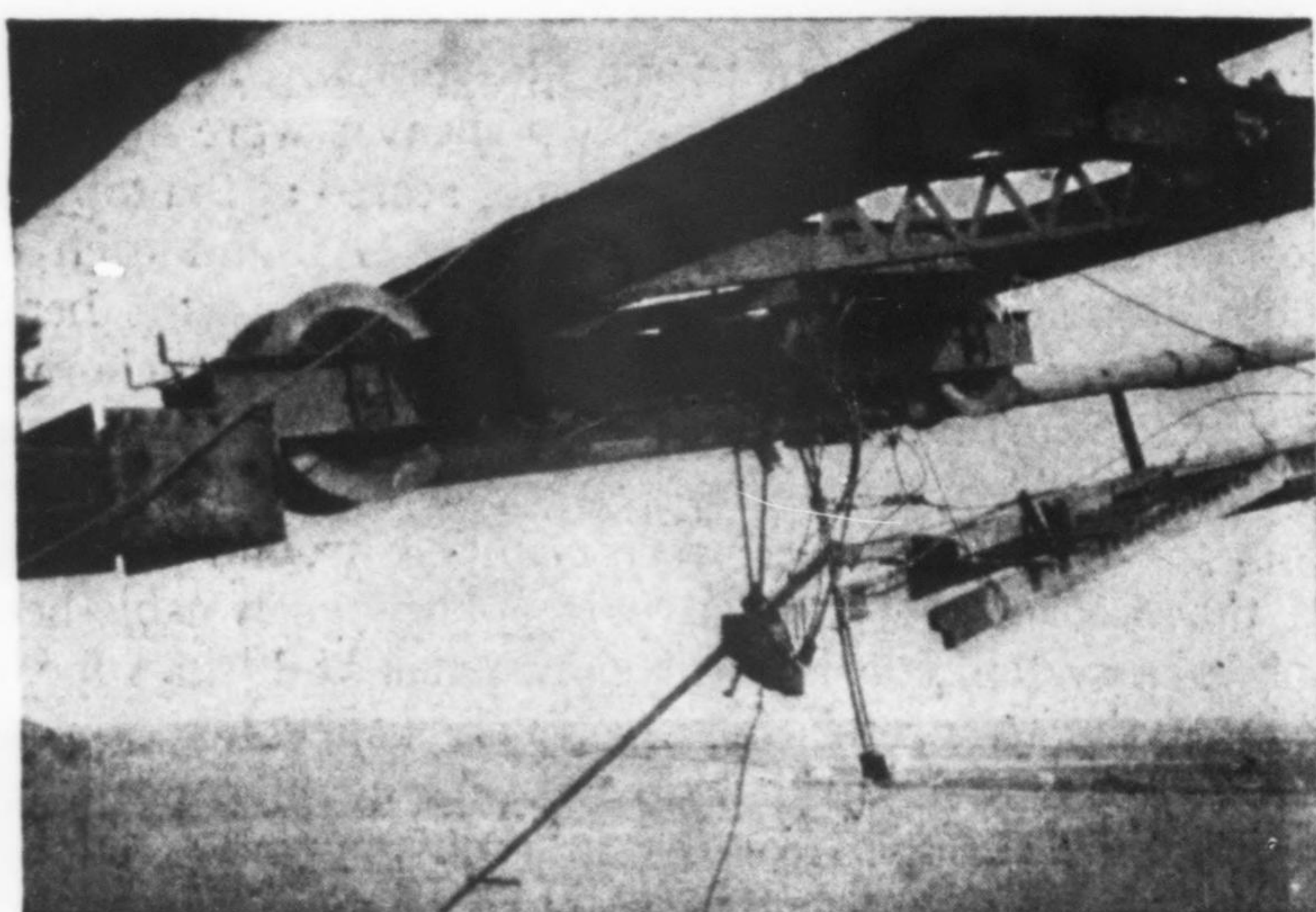
FIG. 5—TRAVELERS AT MOUNT HOPE DESIGNED TO RUN ON CABLES
