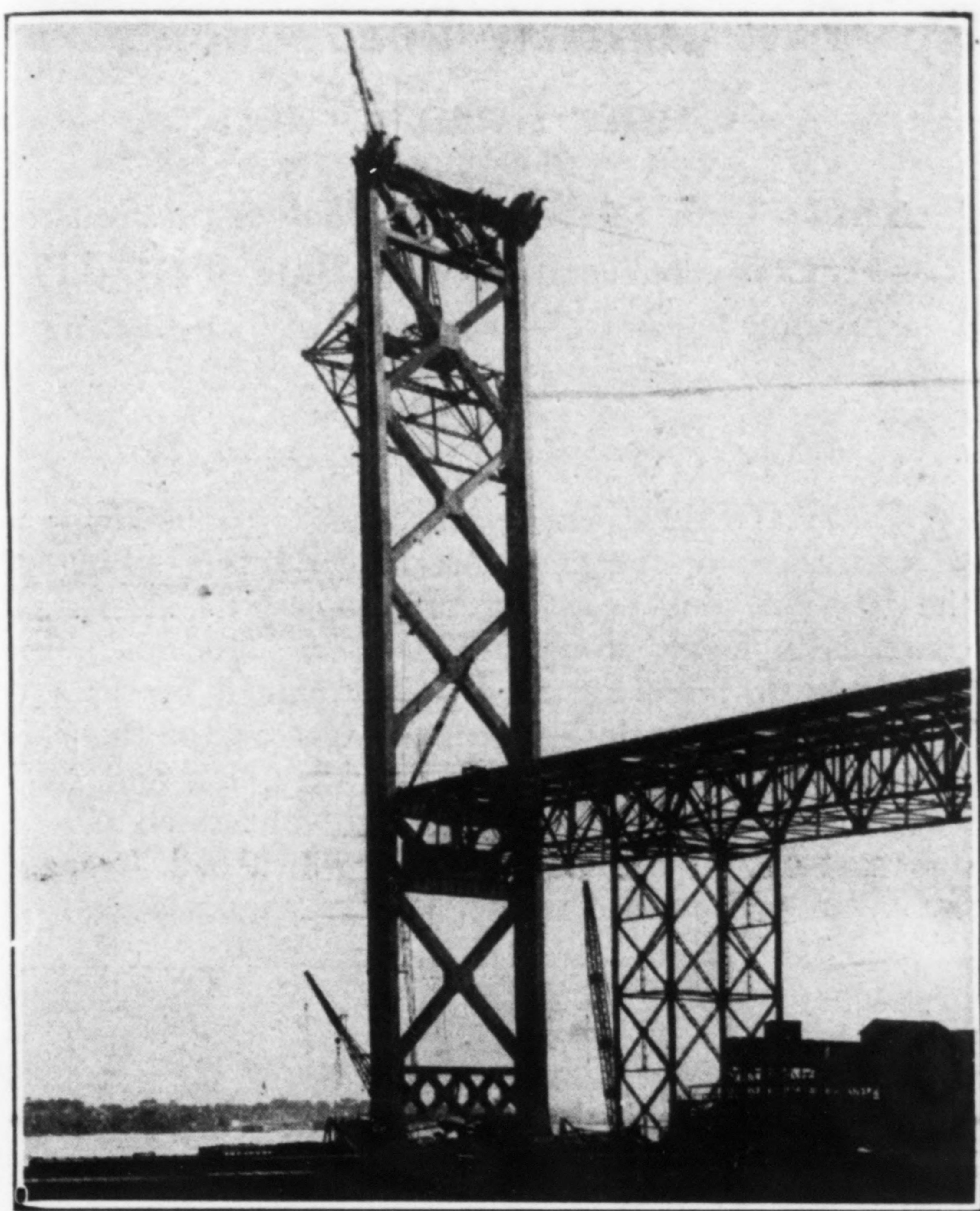
FIG. 8—UNITED STATES TOWER COMPLETE WITH FOOTWALK CABLES IN PLACE
