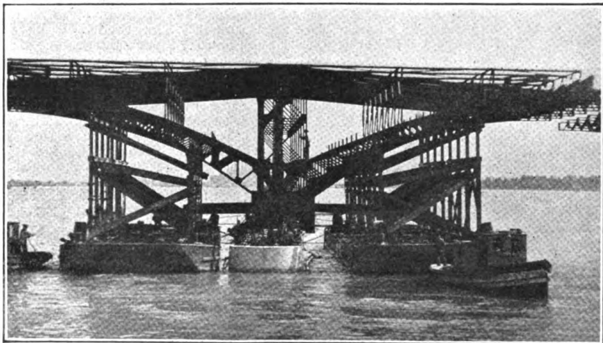
NOVEL STEEL-ERECTION METHOD USED AT BELLE ISLE BRIDGE
