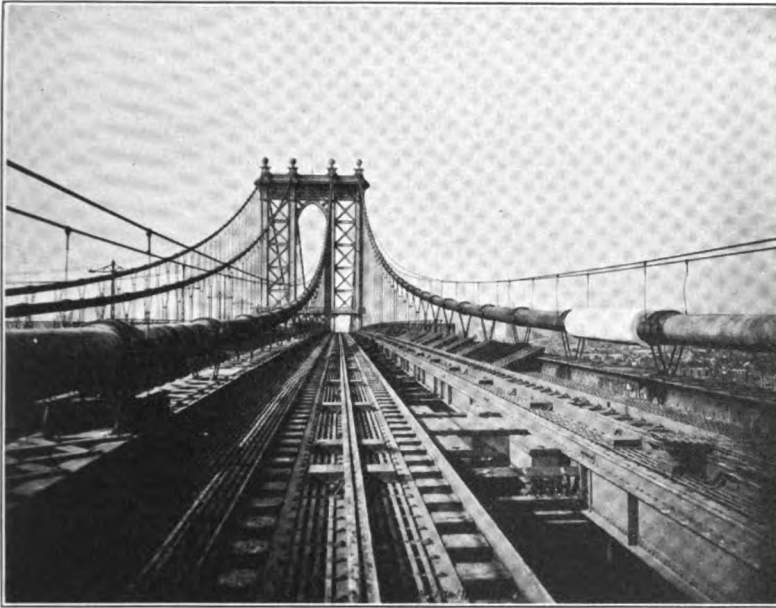
THE MANHATTAN SUSPENSION BRIDGE WITH A MODEL OF THE DELAWARE RIVER BRIDGE CABLE IN PLACE ON THE RIGHT HAND CABLE
