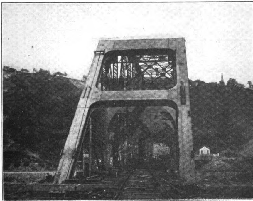
Clairton Bridge: End View of Channel Span, Showing Massive Construction.
