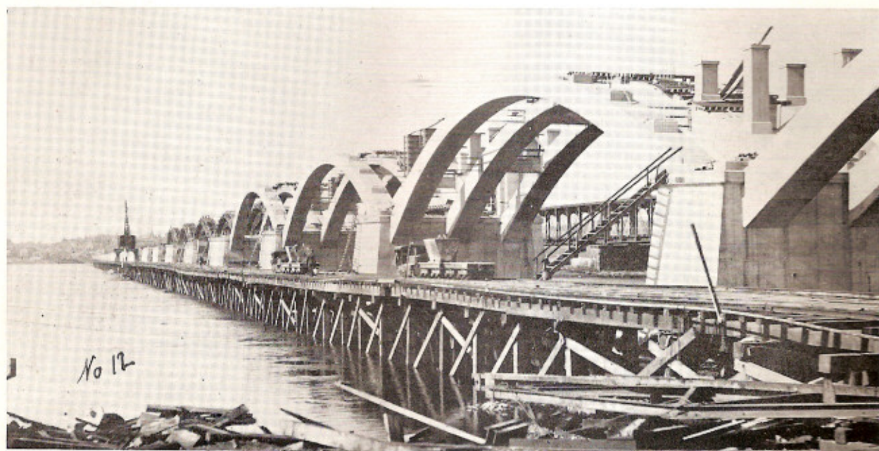
THREE-RIB PARABOLIC ARCHES, TIMBER TRESTLE AND GASOLINE LOCOMOTIVES
