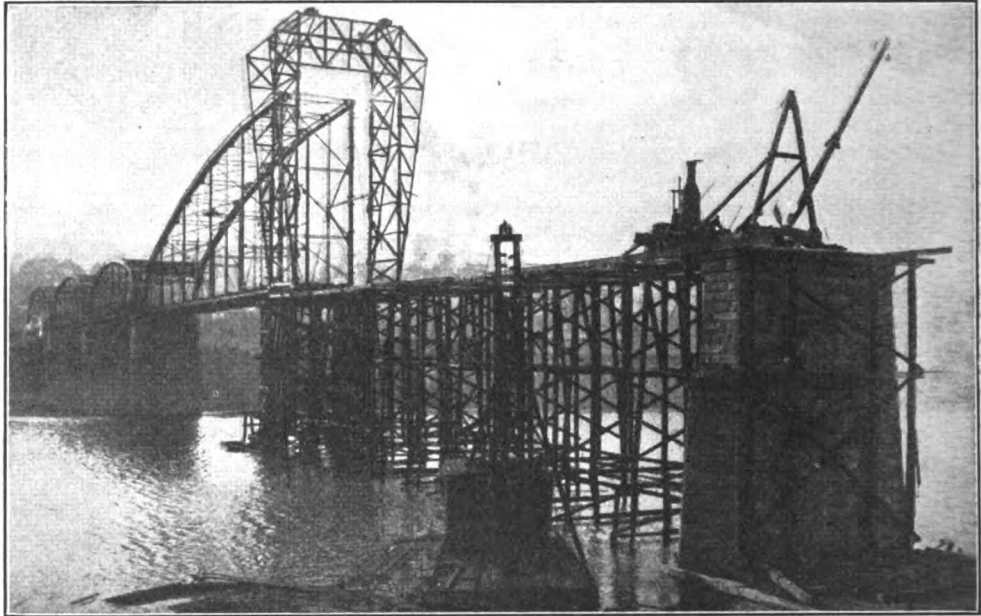
Falsework in Position for Second Half of Webster-Donora Bridge.
