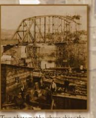
Two photographs above show the construction of the Pennsylvania Truss main span in 1908.
