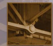
Detail of pinned connection on lower chord of bridge.
