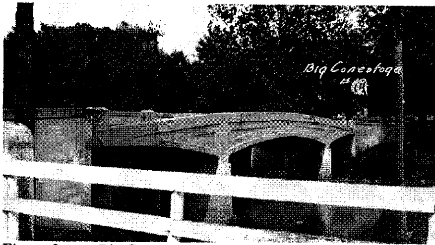
Figure 2. Big Conestoga Creek Bridge No. 12, concrete cantilevered through girder constructed by Paul D. Kauffman in 1917. Source: Lancaster County, Bridge Docket, Lancaster County Engineer's Office, Lancaster, Pa.
