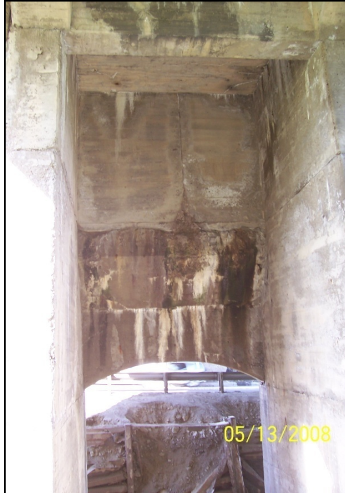
Photograph 17: Deterioration at concrete pier.
