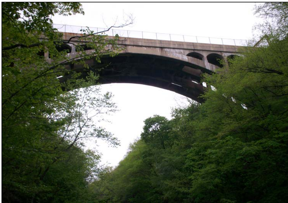
Photograph 2: West elevation of Harrison Avenue Bridge showing Span 2 (spandrel arch) over Roaring Brook Gorge.
