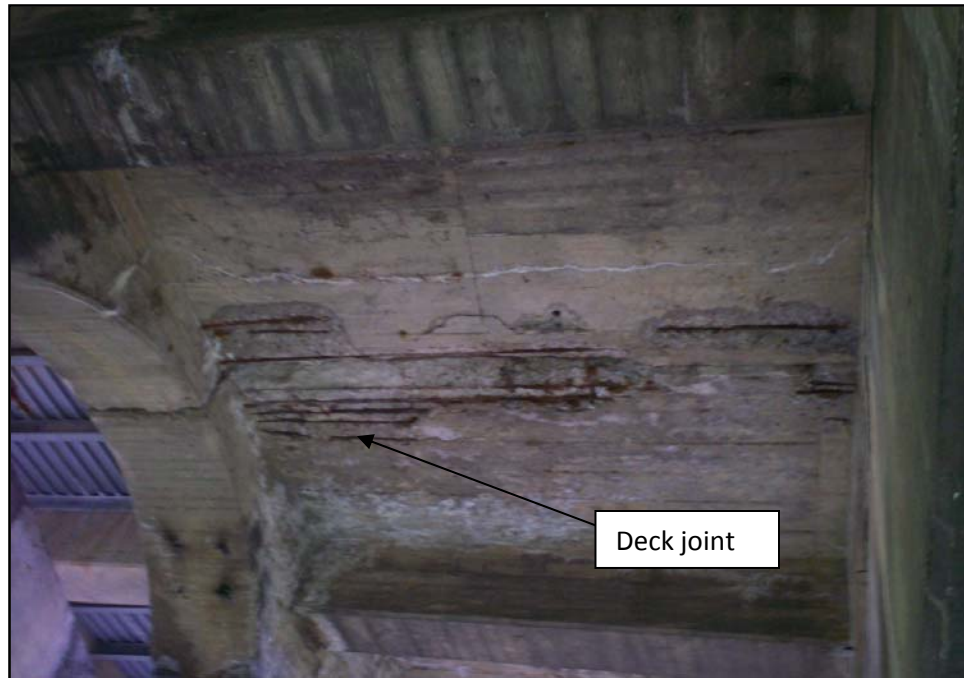
Photograph 11: Underside of deck of Span 2 at joint 2 between ribs 2 and 3, showing deterioration.
