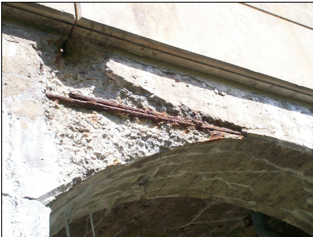
Photograph 14: Exposed reinforcement bars and spalling on the east face of Span 3.
