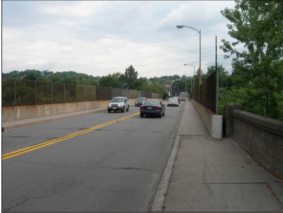
Photograph 7: Deck and bridge railing, view from southeastern corner. The curb-to-curb width of the existing bridge is 30'-0".
