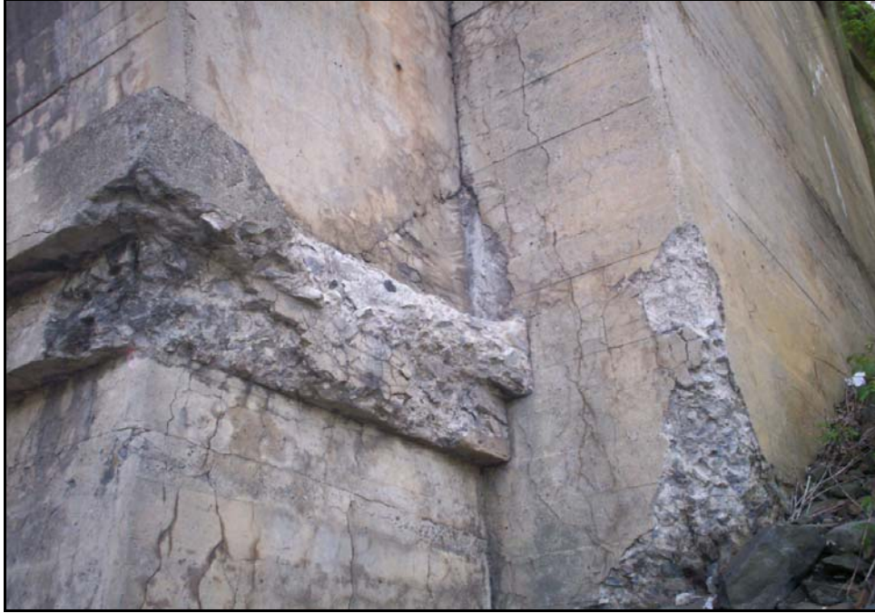
Photograph 15: Deterioration of corner of abutment.
