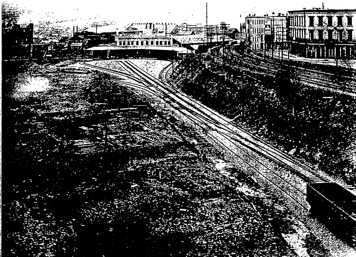
The Scranton terminal and loop track was partly completed during the winter of 1902-1903. Sufficient third-rail had been installed to permit testing of cars as they were received but the southbound mainline track remains incomplete. A temporary interchange track to the DL&W permitted delivery of supplies; it passes through the later site of the station excursion platforms. The DL&W passenger station was a half-mile farther west along Lackawanna Avenue at this time; the present building would be erected to the right six years later.
