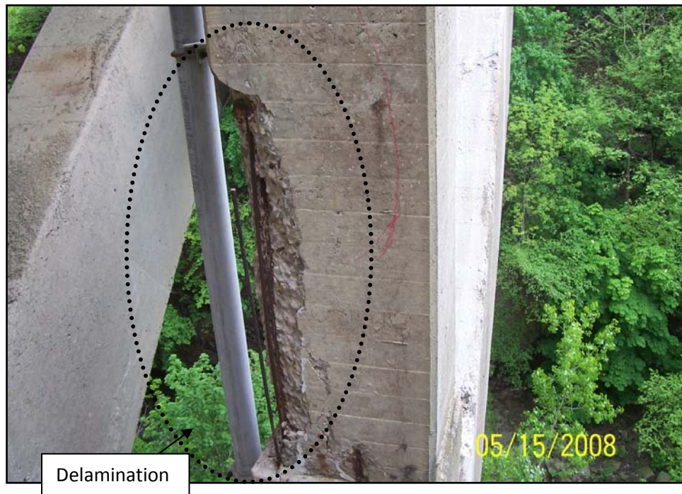
Photograph 12: Loss of concrete at lower portion of column, typical of Span 2.
