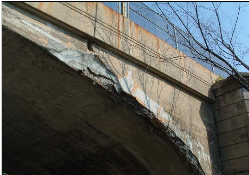
Photograph 10: East face of Span 1, near pier, showing concrete deterioration and repair.
