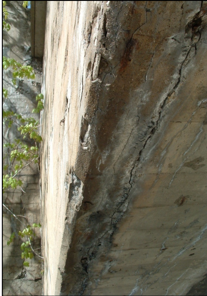
Photograph 8: Delamination of concrete along the east edge of Span 1.
