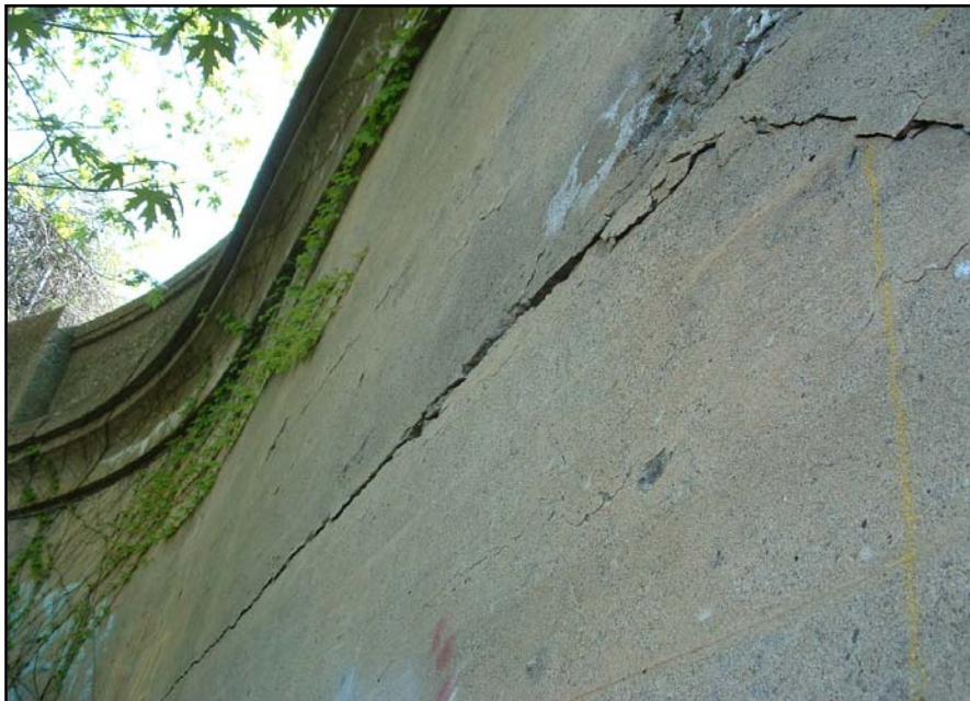
Photograph 16: Displaced construction joint at wing wall.
