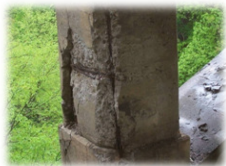
Deterioration of Vertical Spandrel Column in Span 2
