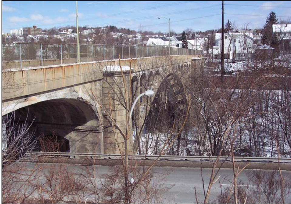
Photograph 1: East elevation of Harrison Avenue Bridge showing Span 1 (barrel arch) and Span 2 (spandrel arch) over Central Scranton Expressway and Roaring Brook Gorge, respectively. Note replacement railing.
