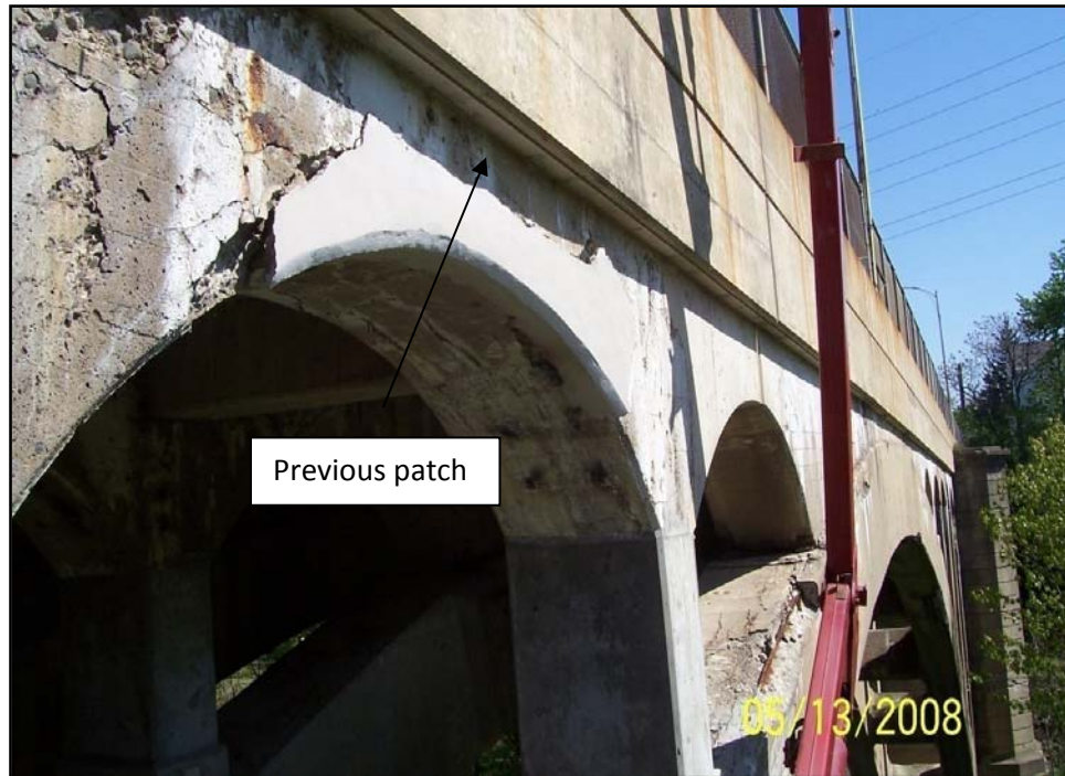
Photograph 13: Span 2, arch beam, showing deterioration and a number of previous concrete repairs.
