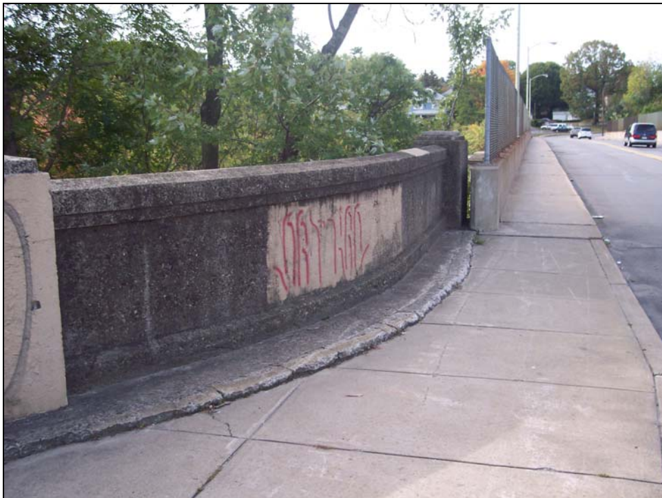
Photograph 6: Northeast corner of Harrison Avenue Bridge showing original railing and 1973 replacement railing topped by protective fence.
