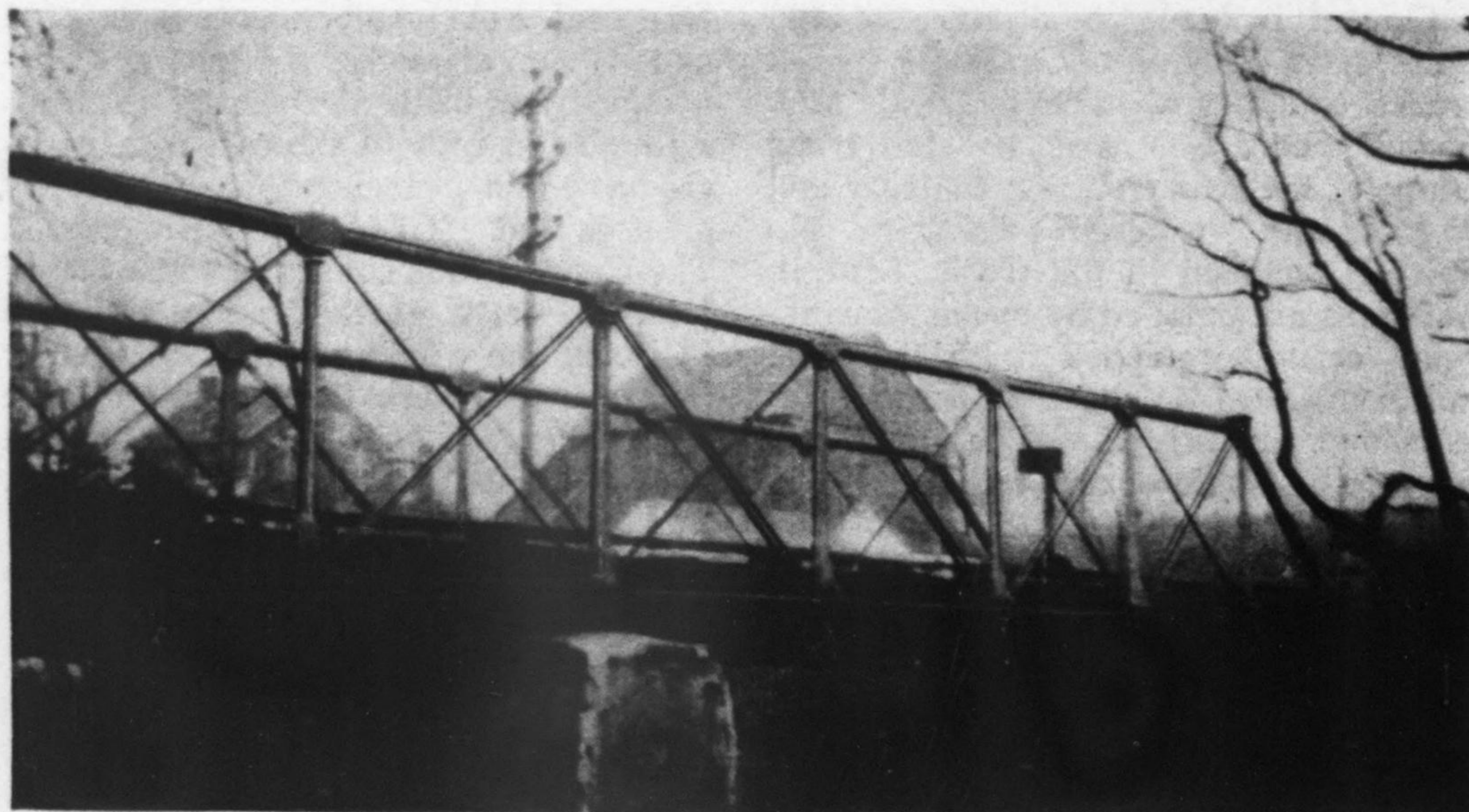
Fig. 4—Continuous-type truss bridge of cast iron in two spans of 52 ft.
