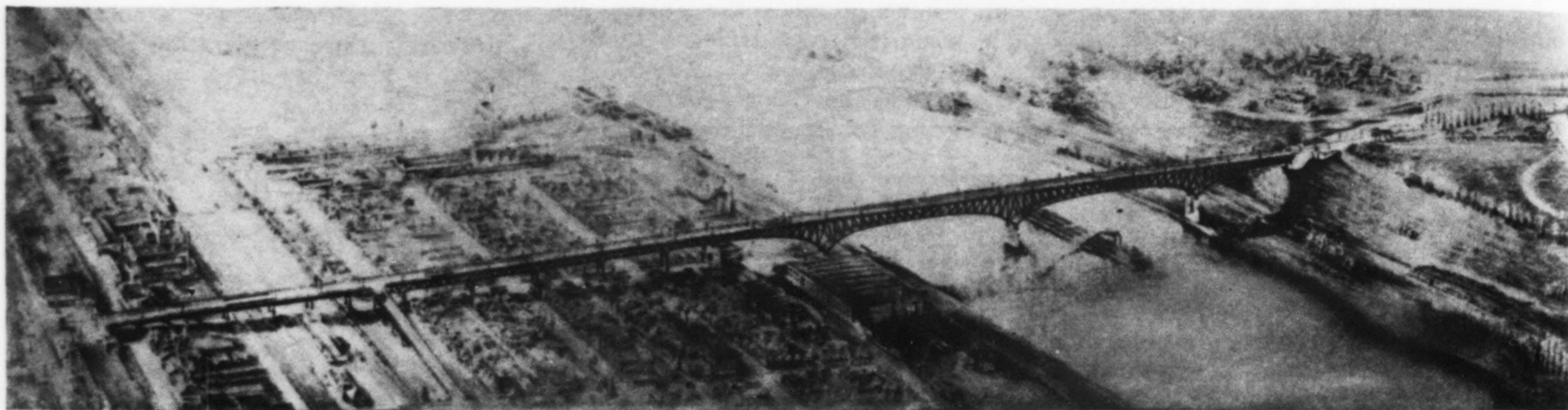
FIG 1—NEW TYPE continuous truss bridge over the Monongahela River between Pittsburgh and Homestead which is statically determinate by virtue of pin jointed rhomboid panels over the intermediate piers. The four span main river bridge comprises one continuous group, while the six spans of trusses in the Homestead approach comprise the second group. Eighth Ave. in Homestead is at the left.
