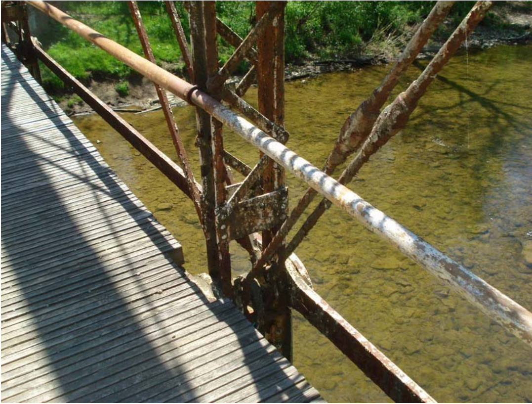
PHOTO 5: BRIDGE RAILING AND PIN CONNECTION
