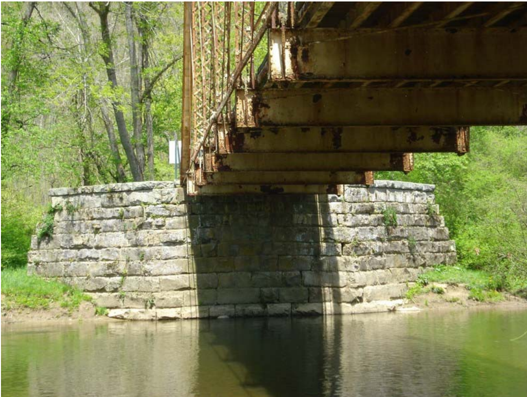
PHOTO 4: FLOORBEAMS, HANGERS, AND ABUTMENT
