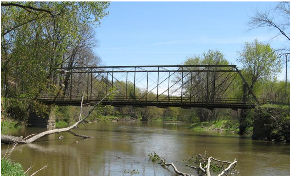
Millers Station Highway Bridge (Source: A&HC 2010)
