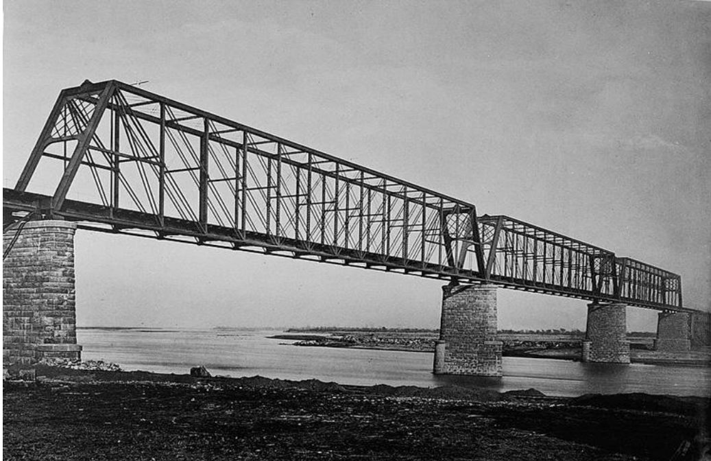
Blair Railroad Bridge (Source: HAER, NE-7-1)
