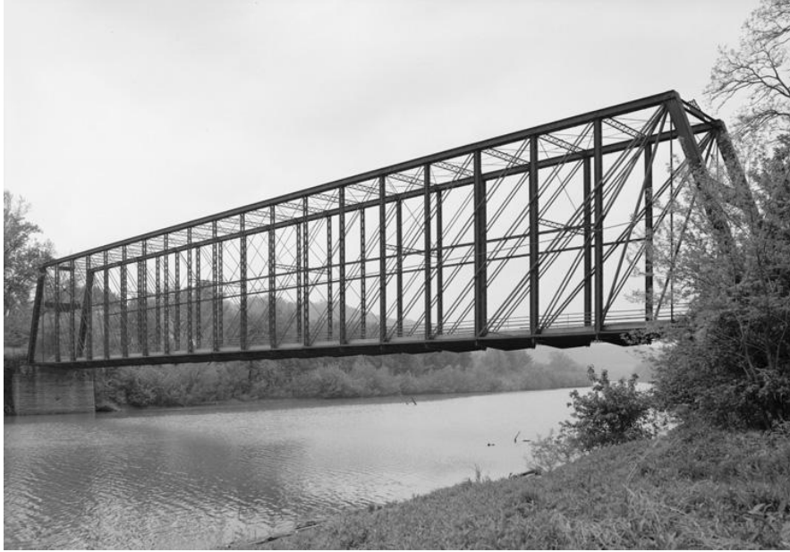
Laughery Creek Highway Bridge (Source: HAER, IN-16-2)
