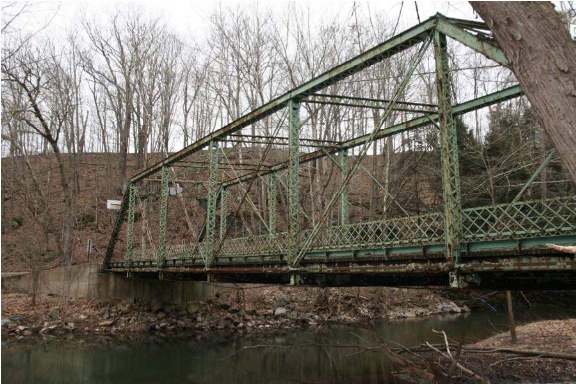
Photograph 14: Overview of the S.R. 2069-001 bridge, looking northwest. The west abutment was replaced in 1975 and will be retained (January 2012).
