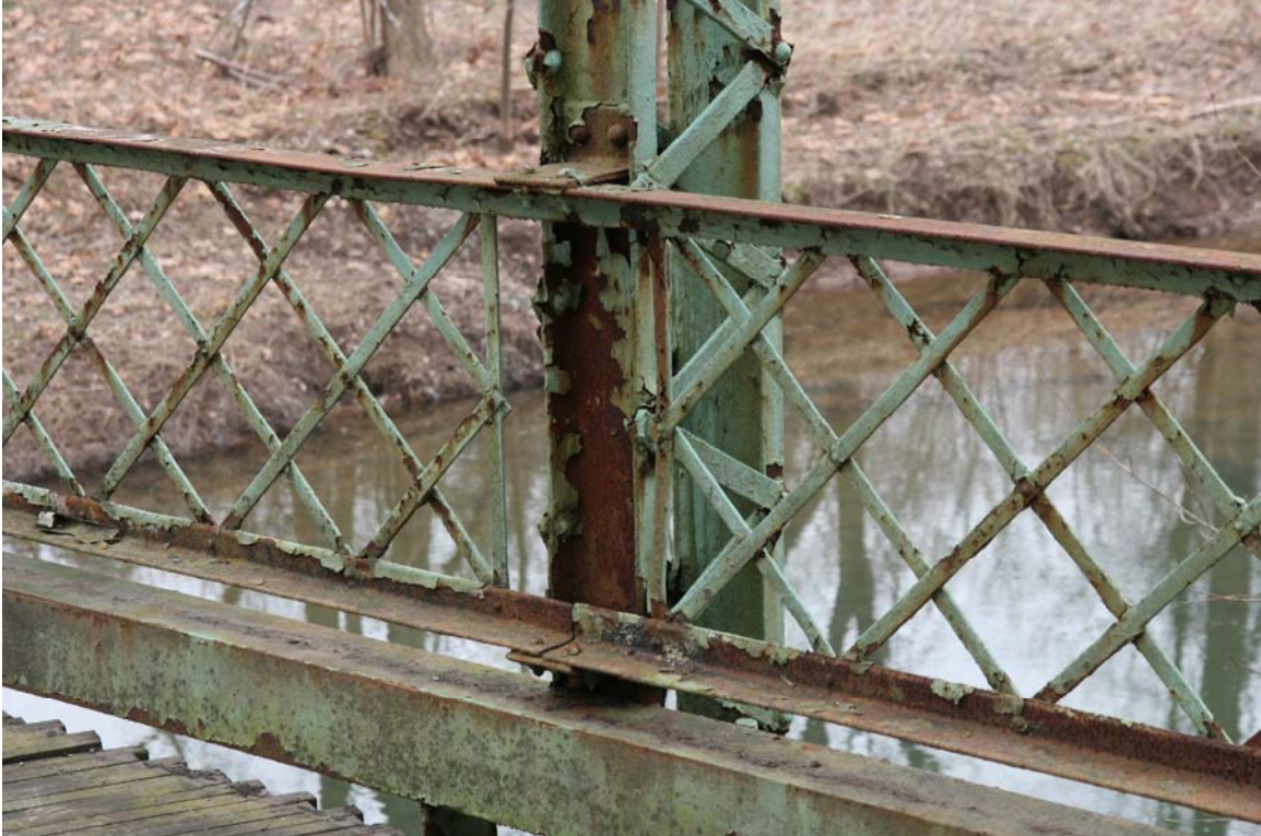
Photograph 12: Detail of the vertical member and railing, looking southeast. The vertical members will all be replaced, and the railing will be replaced in-kind with a new W-beam railing (January 2012).
