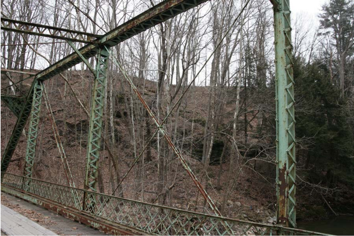
Photograph 11: Detail of the north side of the S.R. 2069-001 bridge, looking northwest, showing the deteriorated vertical and diagonal members, which will be replaced (January 2012).
