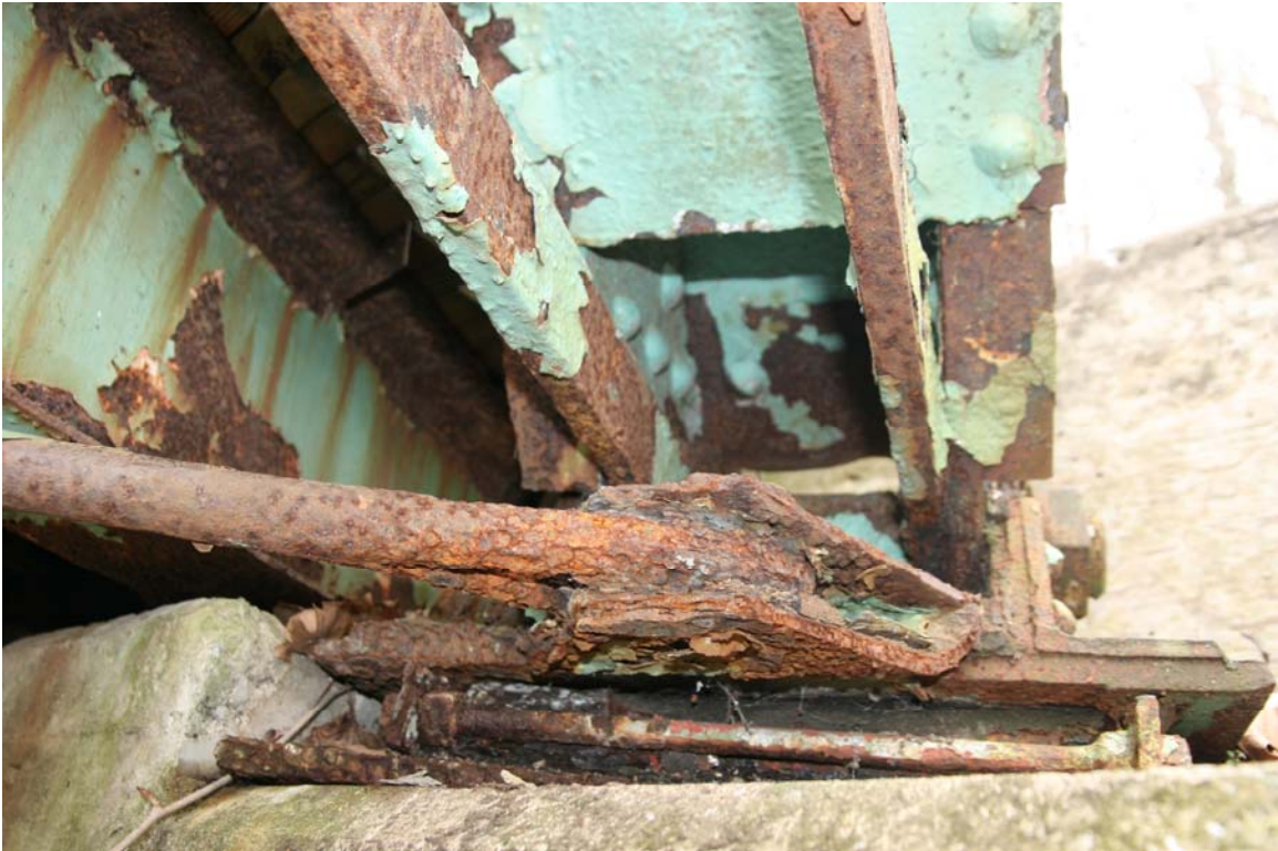
Photograph 10: Detail of the deterioration at the connection of the lower chord, lower lateral bracing, and east portal of the S.R. 2069-001 bridge, looking southwest (January 2012).
