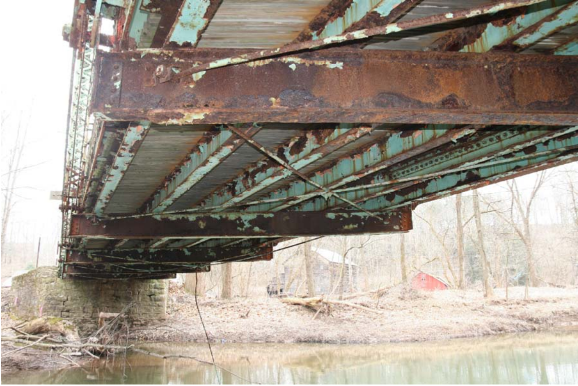
Photograph 7: View underneath the S.R. 2069-001 bridge, looking northeast, showing the deterioration of floor beams, stringers, and lower lateral bracing (January 2012).
