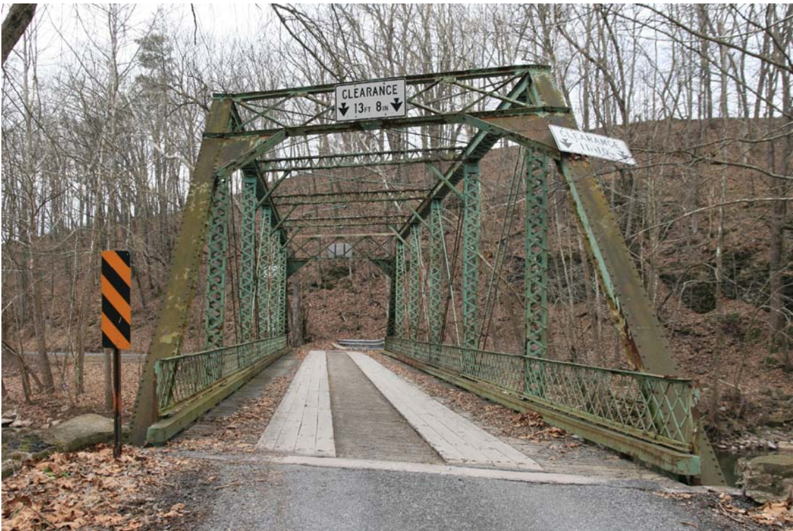
Photograph 6: View looking west toward the east portal of the S.R. 2069-001 bridge. The portal, top struts, and upper lateral bracing will be retained through minor repair work. The previously repaired timber deck will be replaced with a galvanized steel open deck (January 2012).
