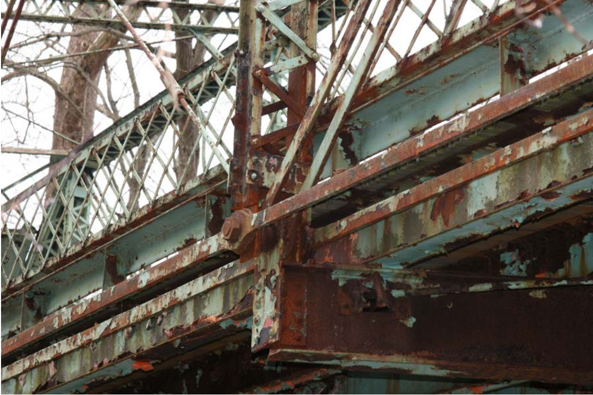
Photograph 9: Detail of the lower connection of vertical members and floor beam, looking southeast. The floor beams, lower chord, and vertical members will all be replaced. The eye bars will be replaced in-kind (January 2012).
