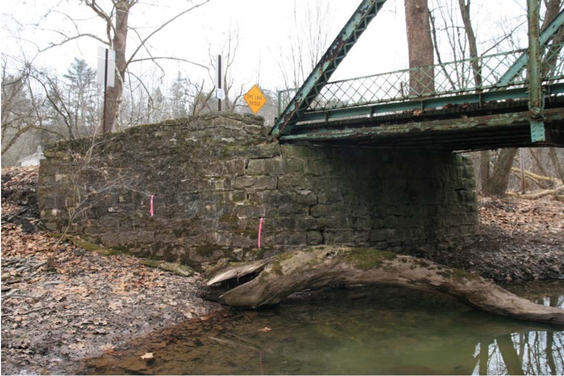
Photograph 13: Detail of the east abutment, which will be retained, looking southeast. The stone will be repointed, drainage will be placed behind the abutment, and a new concrete cap will be applied (January 2012).
