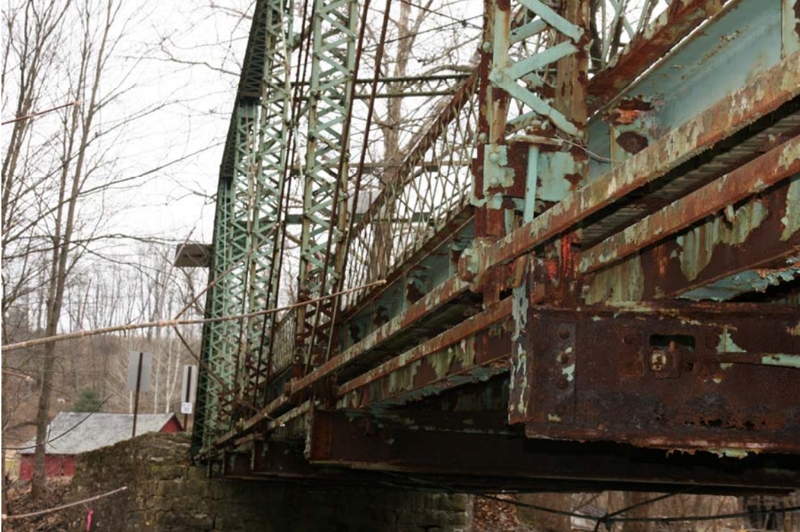
Photograph 8: Detail of the north side of the S.R. 2069-001 bridge, looking east, showing the deterioration of the floor beams, lower chord, and vertical and diagonal members (January 2012).
