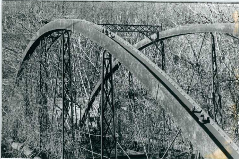
View of bridge, looking northwest. Note truss and joints.
