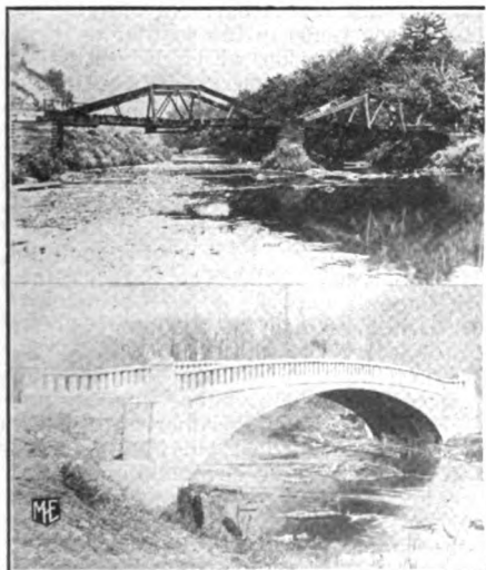
No. 12. Old and new bridges over Elk Creek, near Ridgway, Pa. Concrete bridge cost $5,300.
