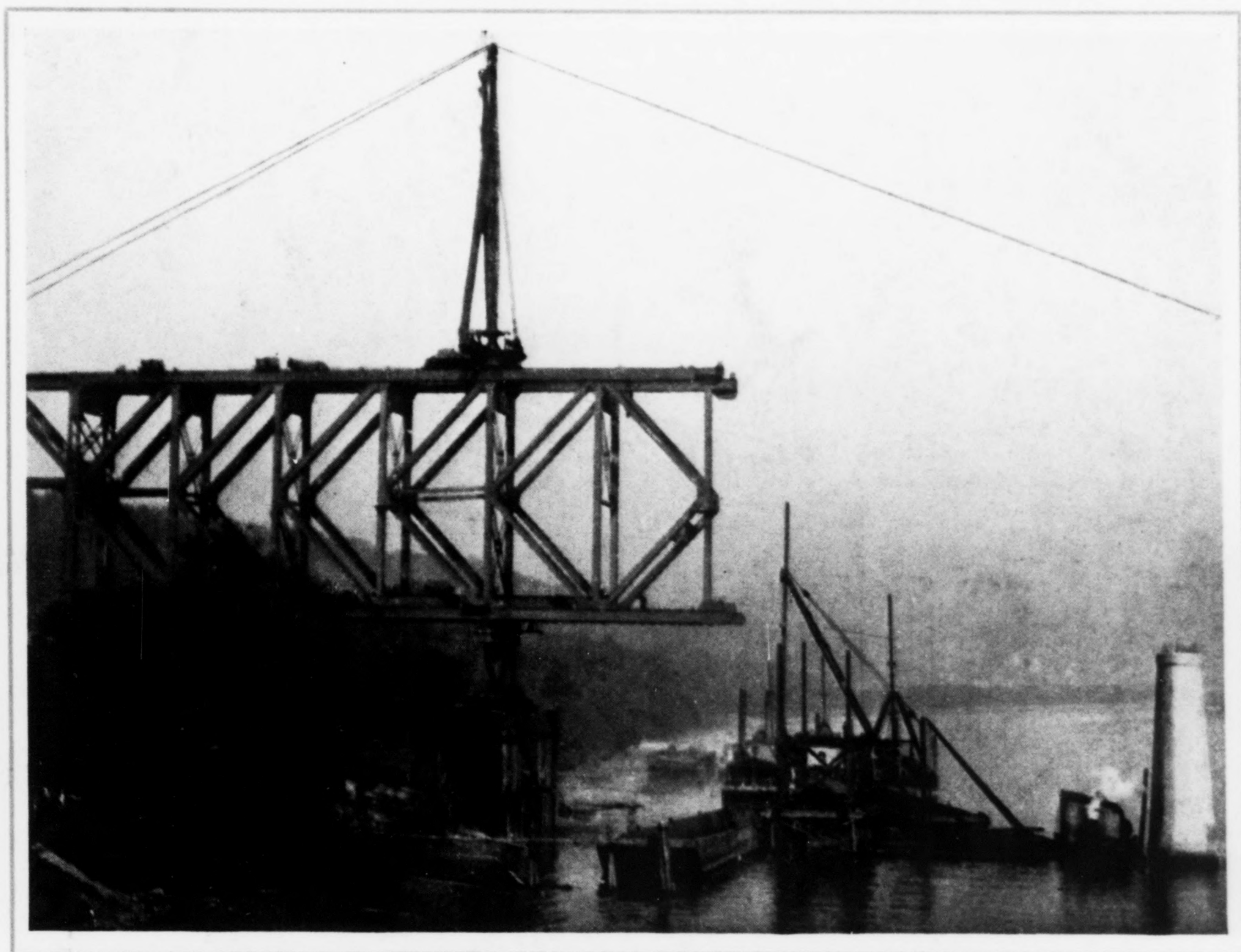
Erecting K-braced trusses of Pittsburgh & West Virginia Ry. bridge over the Monongahela River
