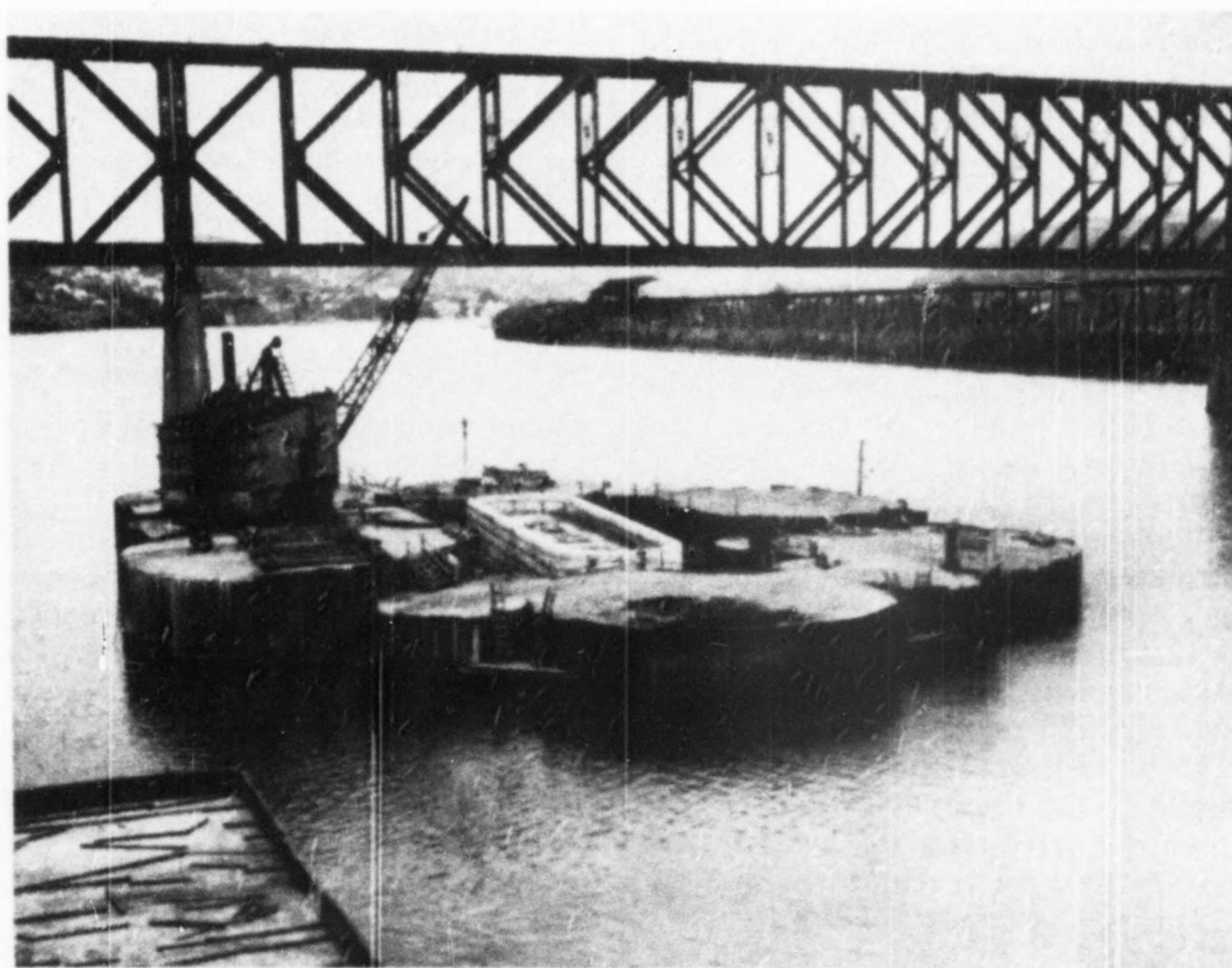
NEW HIGHWAY BRIDGE —Cellular steel sheetpile cofferdams were used by the Dravo Corp., Pittsburgh, in building the two main river piers for a 2,000-ft, four-lane highway bridge across the Monongahela River at Belle Vernon, Pa. The bridge is a key structure on a road to connect the Pennsylvania Turnpike, at New Stanton, with Route 40, at Washington, Pa., enabling Turnpike-Ohio traffic to bypass Pittsburgh. Underwater portion of each main river pier has concrete shafts embedded in rock 70 ft below water level. Concrete distribution block 89x24x38 ft rests on the shafts and supports concrete columns on which the structural framework will rest. Normal channel clearance will be 431x75 ft.
