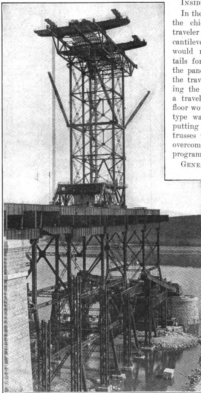
FIG. 1. THE QUEBEC BRIDGE TRAVELER IN WORKING POSITION
