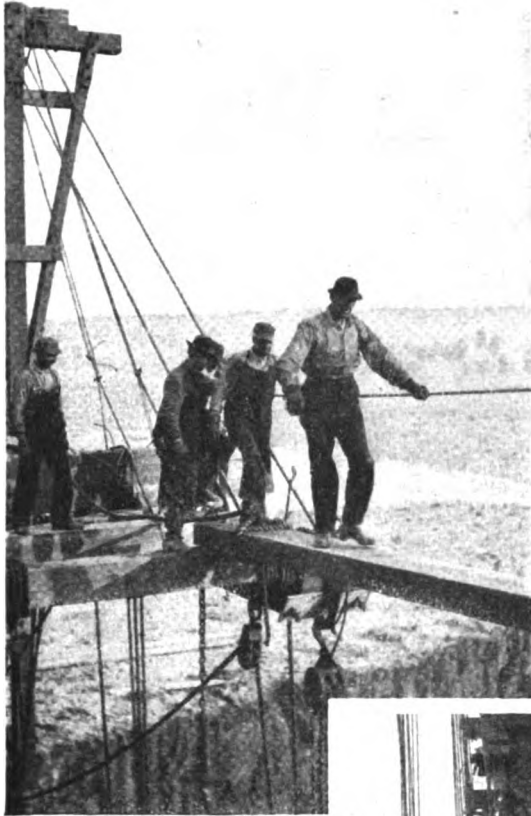
Two views of the Crooked River Bridge during construction. The river runs through a gorge 350 feet deep. In the accompanying article, Mr. Modjeski tells how the men became so careless of danger that they would "coon" across a 30-foot gap on a 4-inch pipe. Walking a substantial plank, as they are doing here, seems quite risky enough
