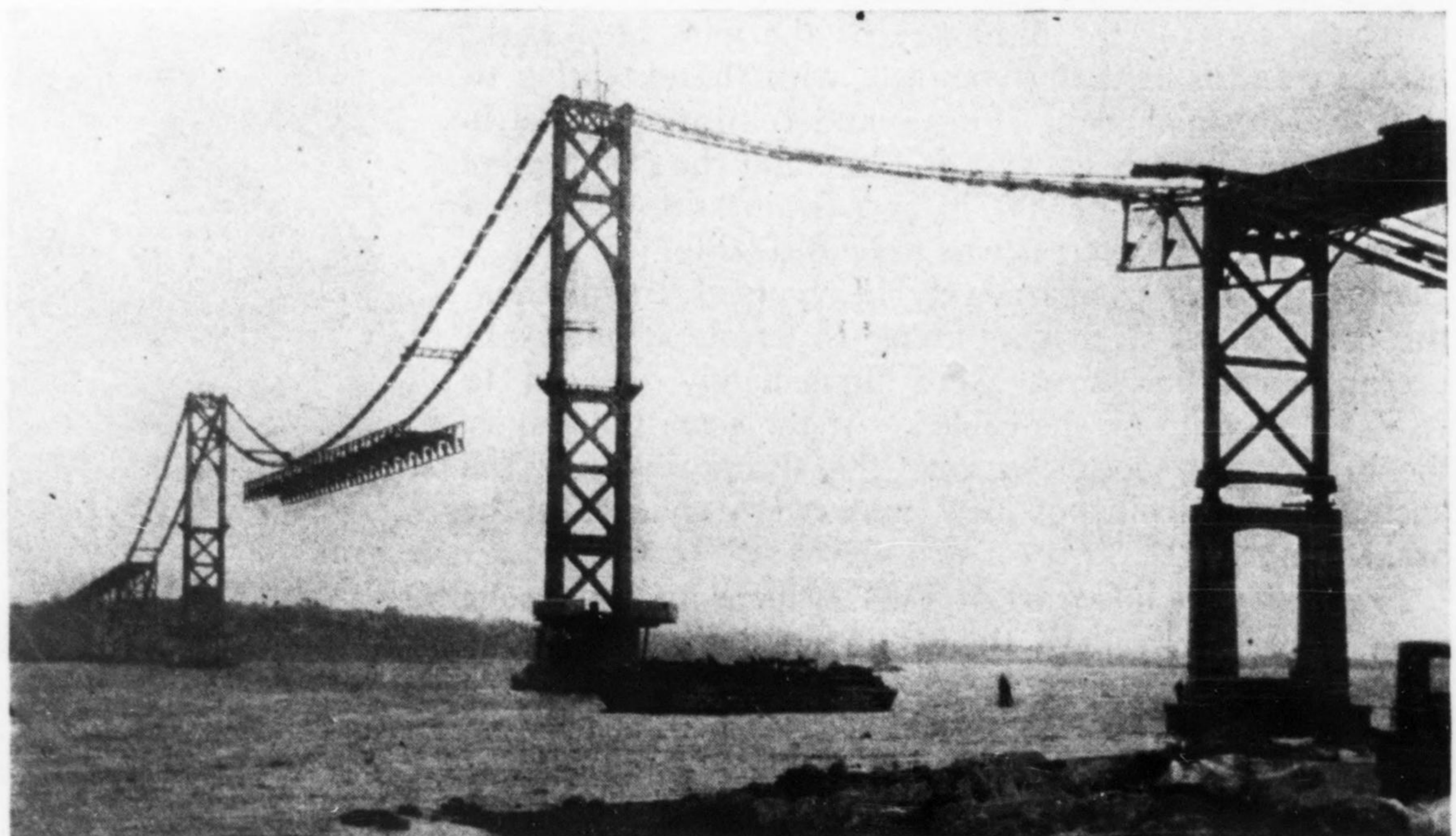
FIG. 6—DISMANTLING TRAVELERS WORKING AWAY FROM MAIN TOWERS, MOUNT HOPE
