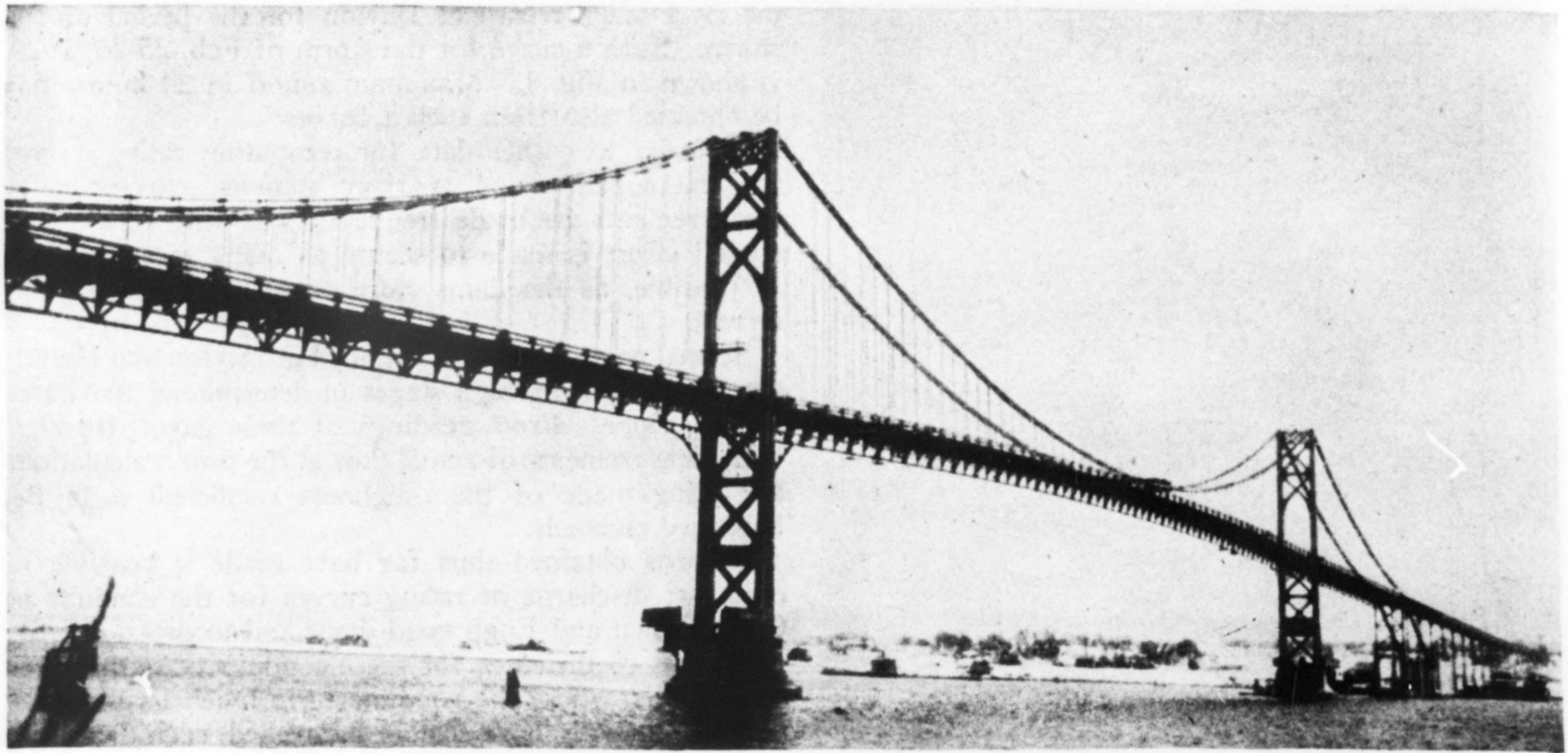
FIG. 1—THE MOUNT HOPE BRIDGE ON FEB. 23 JUST AFTER DISCOVERY OF BROKEN WIRES Preparations were under way for placing concrete floor slab.
