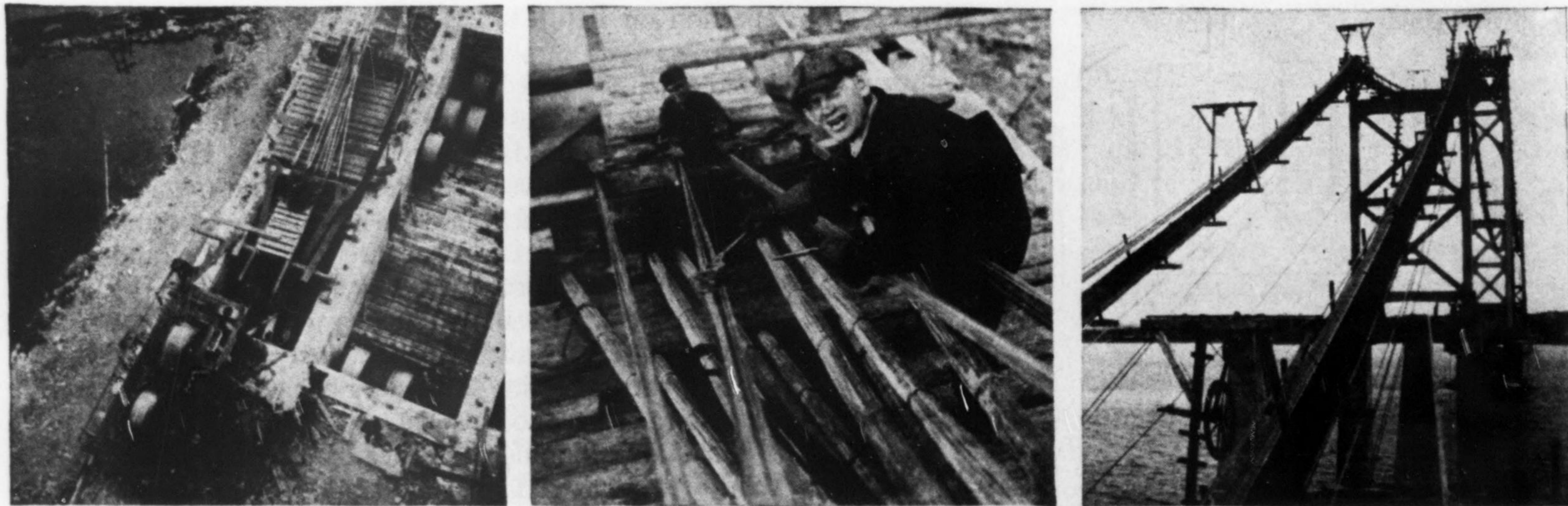
FIG. 5—THREE VIEWS OF THE CABLE-SPINNING OPERATIONS ON THE MOUNT HOPE BRIDGE
