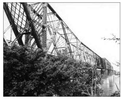
Significant under Criterion A for role in expanding rail traffic between South and Midwest, under Criterion B due to Morison's close involvement with the bridge project, and under Criterion C as Morison's most important bridge design and as an innovative cantilevered continuous truss bridge.
