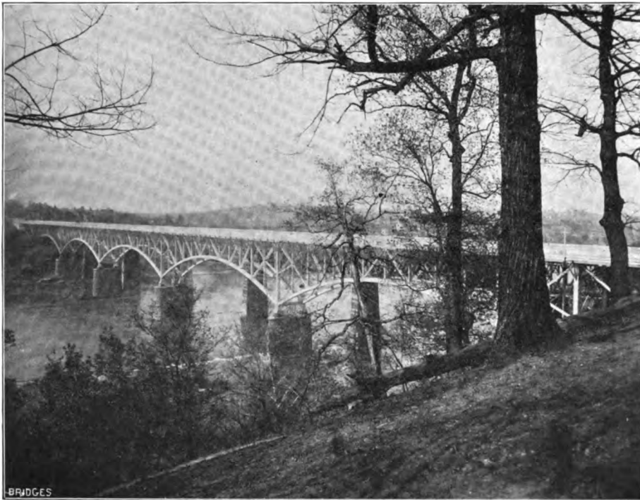
FIG. 18—KNOXVILLE ARCHED CANTILEVER.
