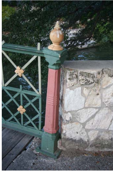
Photo 5: Detail of ornamental railing end panel and end post at southwest corner
