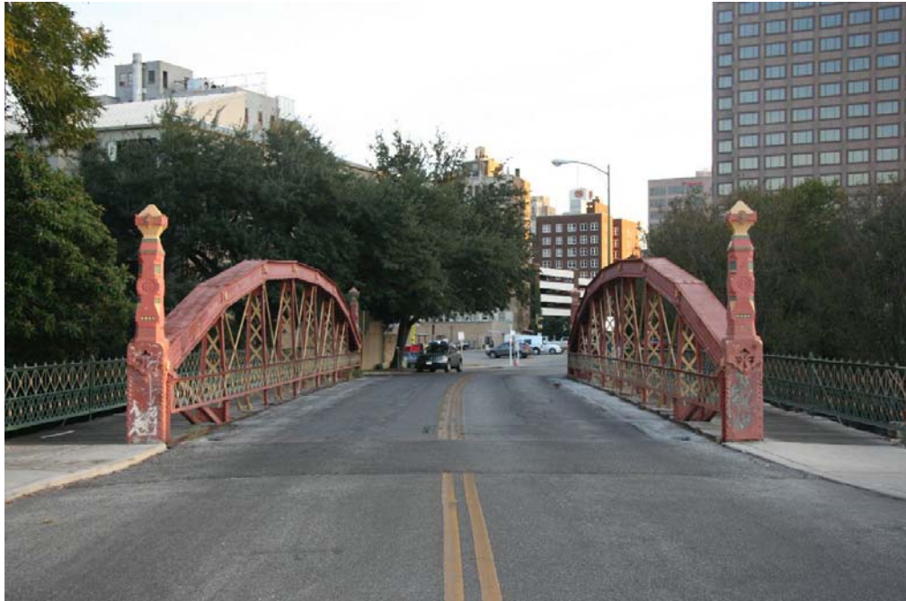
Photo 2: Deck view, facing south
