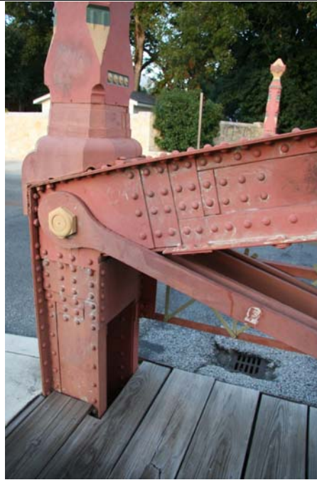
Photo 3: Detail of upper chord pin connection at end post, exterior view
