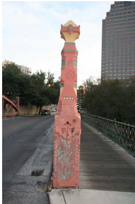
Photo 4: Detail of truss ornamental end post at northwest corner
