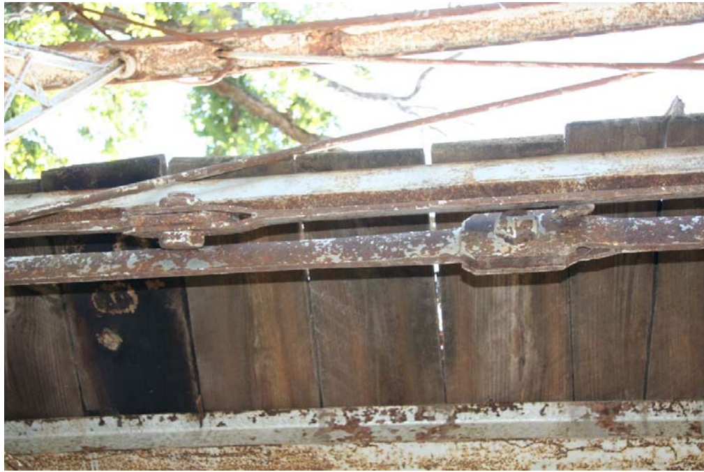
Photo 5: Detail of lower chord end-to-end pinned connection
