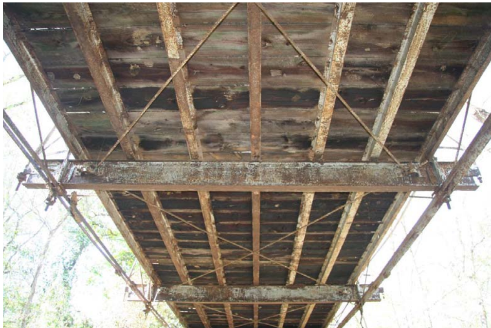
Photo 6: Detail of underside of truss, facing west
