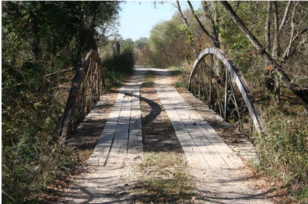
Photo 2: Deck view of east portal, facing west
