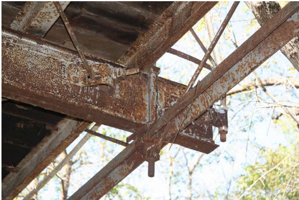
Photo 4: Detail of lower chord connection with floor beam
