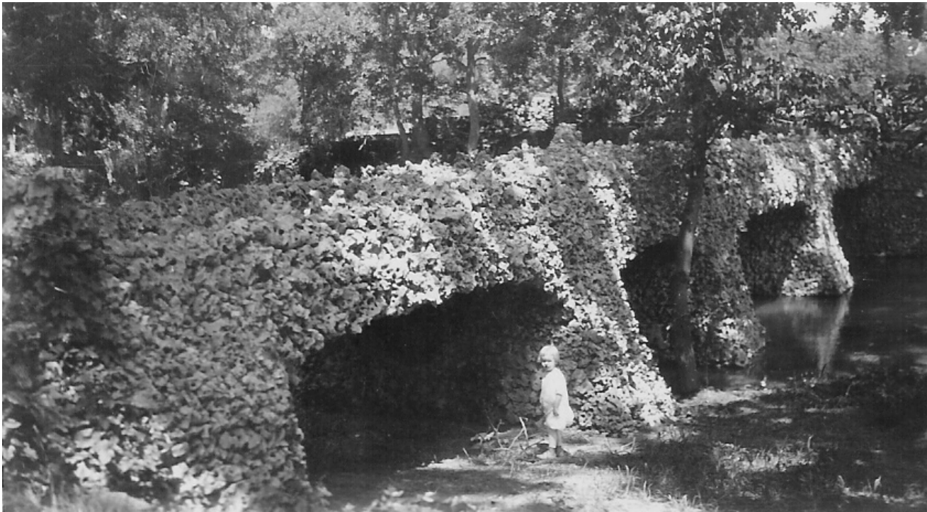
Figure 14. Madarasz Park bridge
