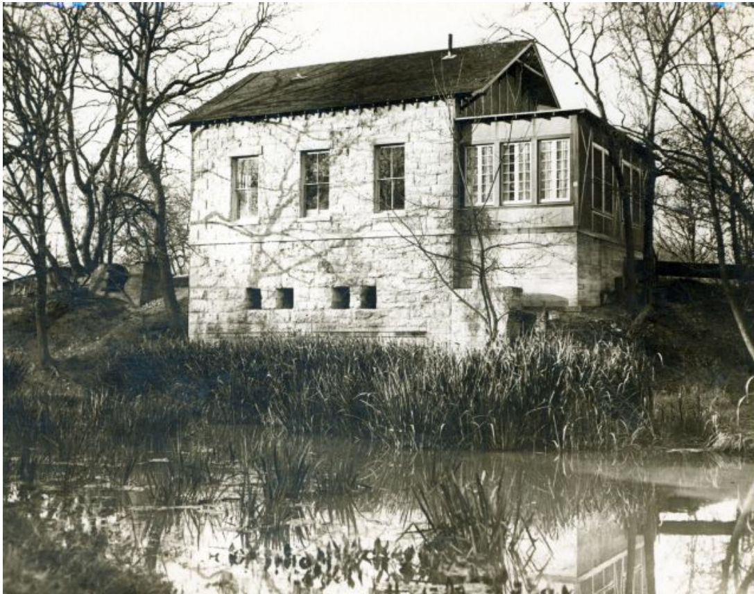
Figure 3. Lower pump house
