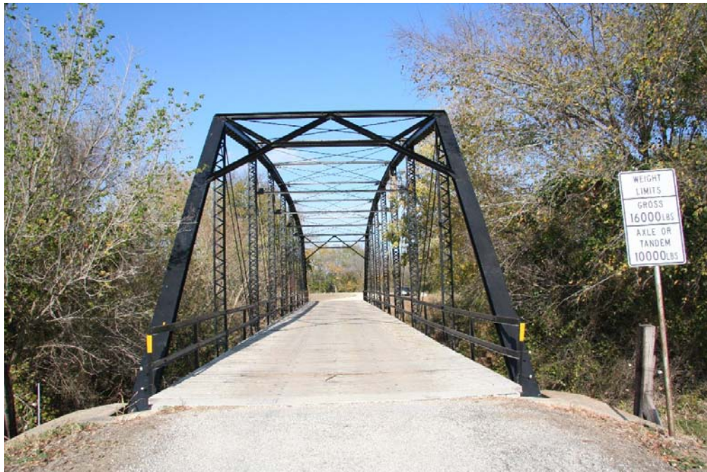
Photo 4: Overview of deck and approach roadway; view facing north
