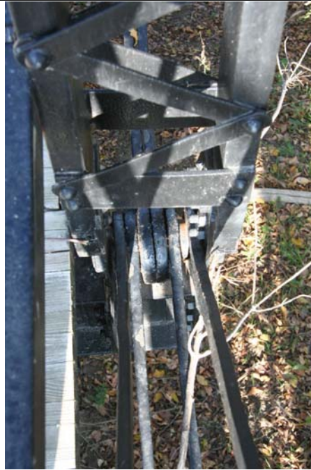
Photo 3: Detail of primary truss connection at lower chord and vertical
