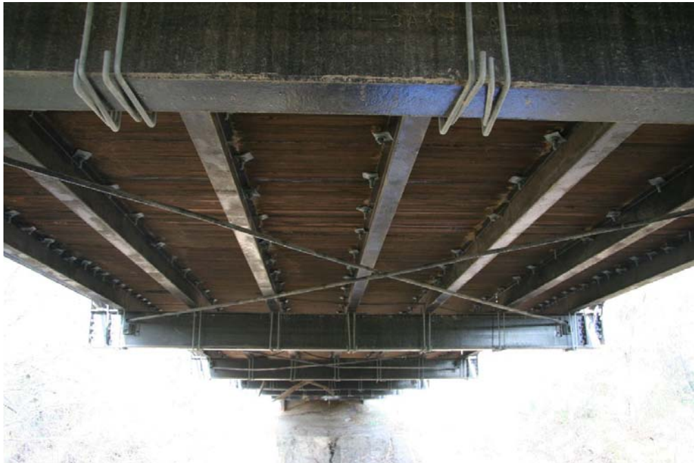
Photo 6: Underside of truss; view facing north
