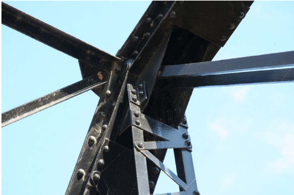
Photo 2: Detail of primary truss connection at top chord and end post
