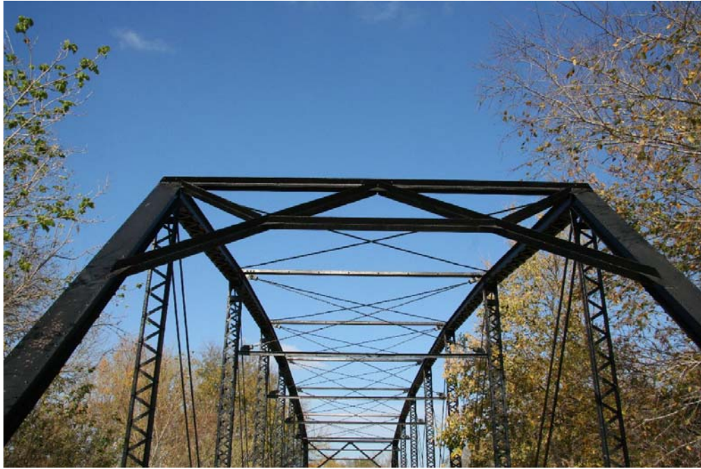
Photo 5: Detail of portal, lateral, and sway bracing; view facing north
