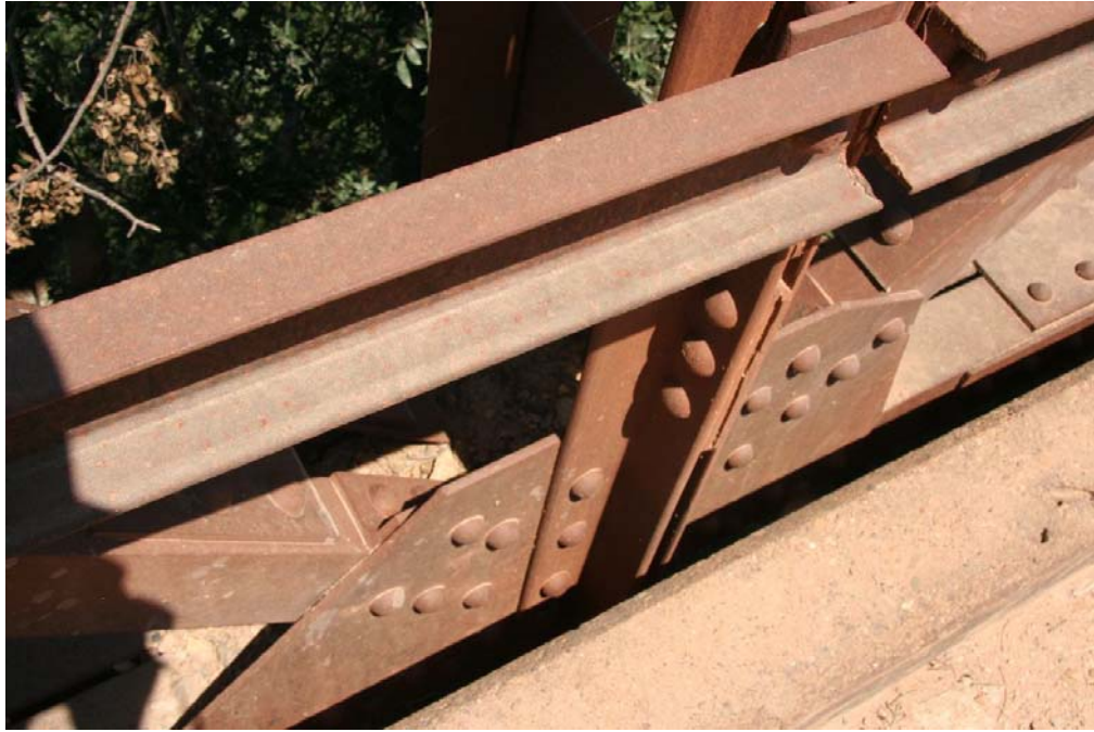
Photo 5: Detail of riveted gusset plate connection at bottom chord
