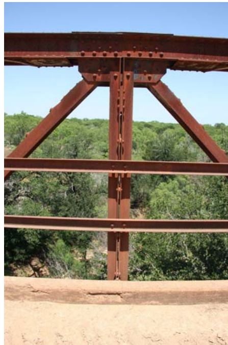
Photo 4: Detail of riveted gusset plate connection at top chord
