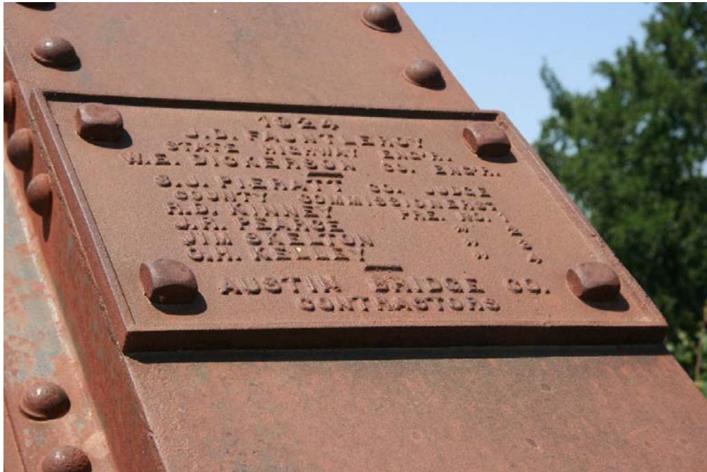
Photo 6: Detail of builder's plate
