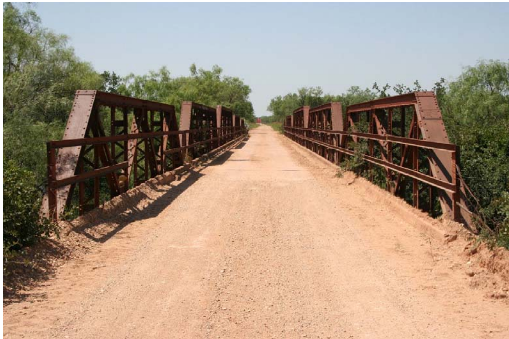
Photo 2: Deck view of bridge facing west
