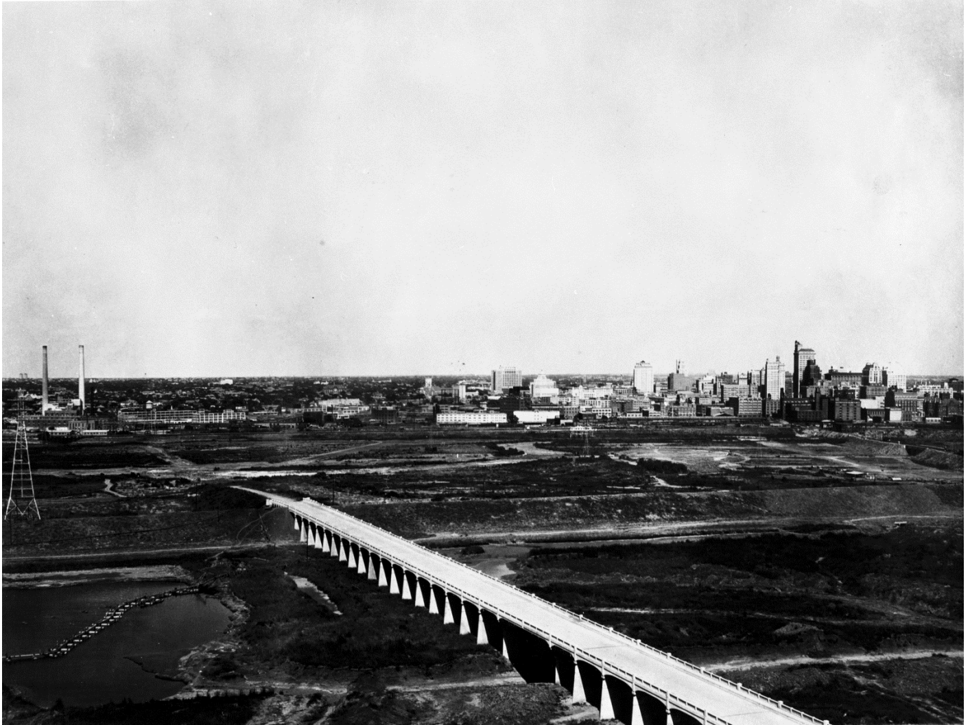
Lamar-McKinney Bridge under construction, c.1930 Source: Dallas Public Library
