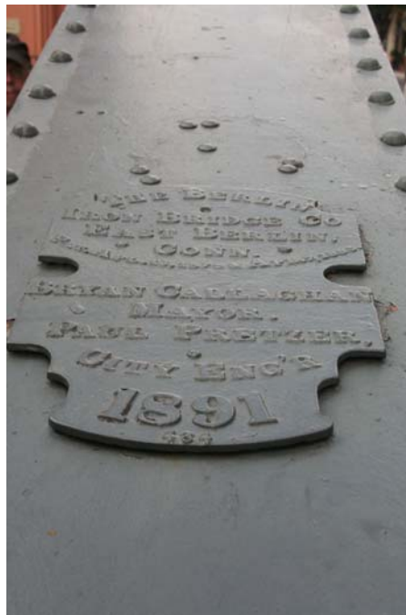
Photo 6: Detail of builder's plate
