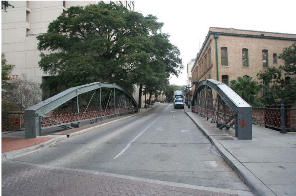
Photo 2: Deck view, facing east
