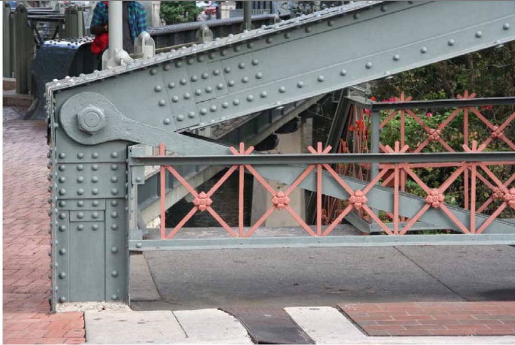
Photo 3: Detail of pin connection joining top chord, bottom chord, and lenticular end post
