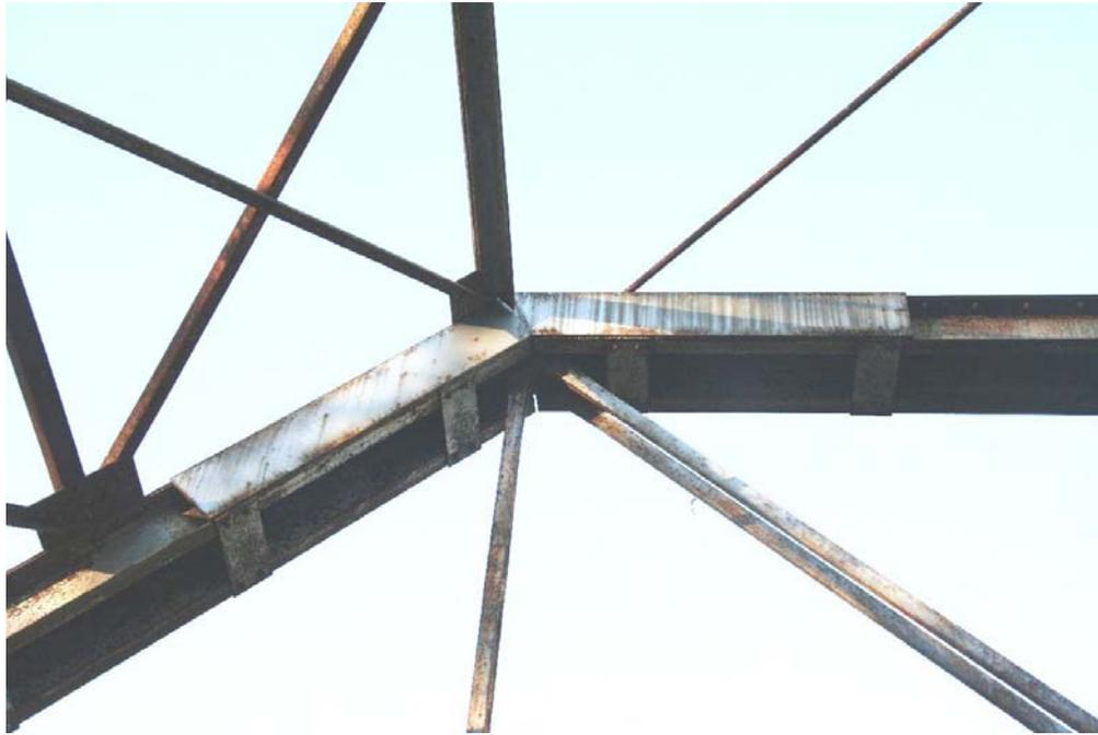
Photo 5: Detail of welded plates at upper chord connections
