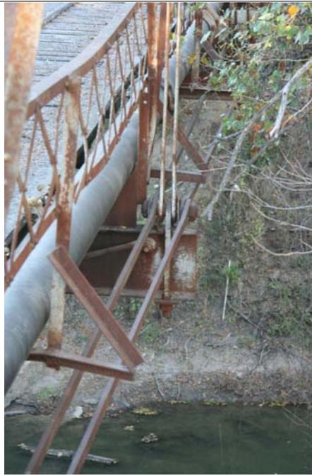
Photo 3: Detail of primary connection at bottom chord
