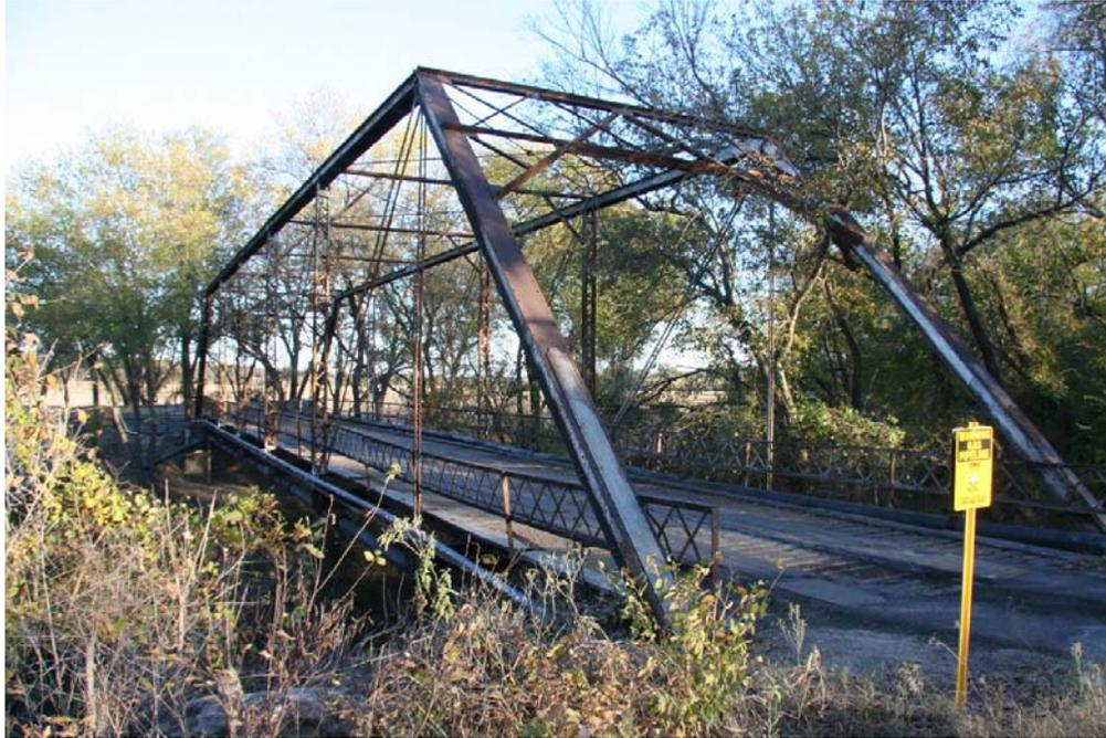
Photo 1: Elevation of one-span, pin-connected Pratt through truss, a rare survivor of a once common truss type in the state; view facing southeast
