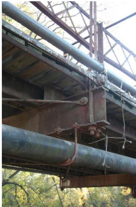
Photo 6: Detail of utility lines attached to the bridge
