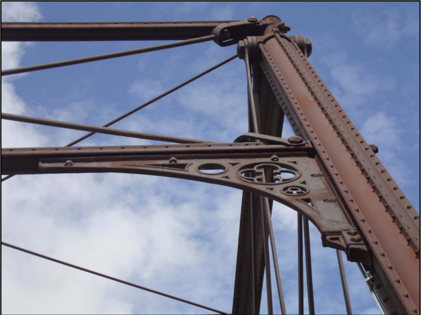
Figure 6: Portal bracing with quatrefoils and Phoenix column. (Photo by Pat Sparks)
