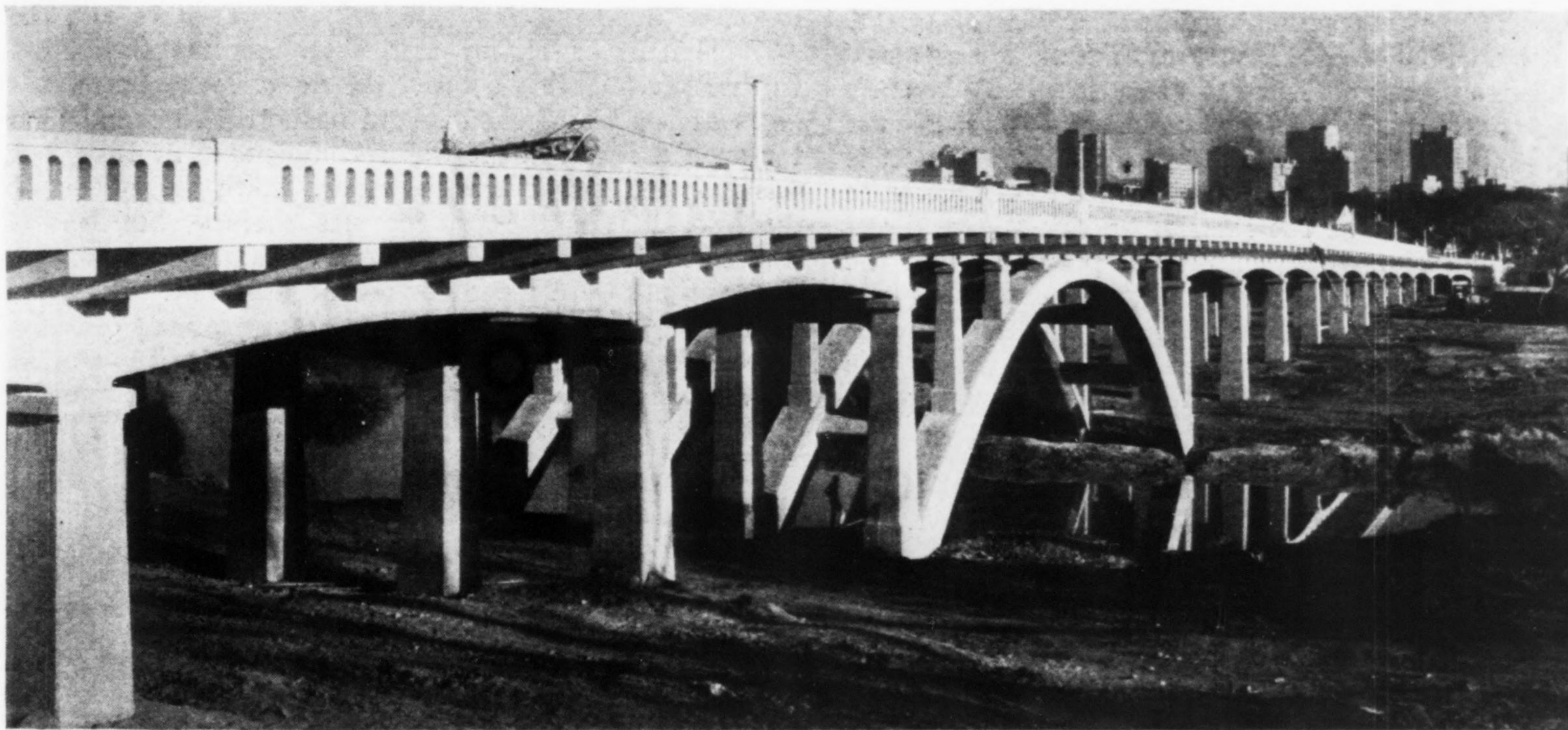
Royal Street Bridge in Fort Worth, Tex., presents a pleasing combination of arch and girder spans.
